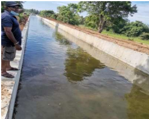
Figure 6-29: D1 North Canal Lining in PSS
