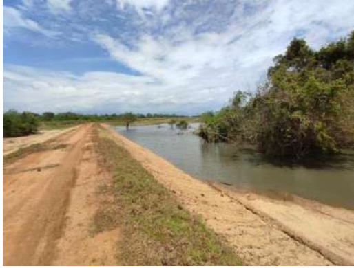
Figure 5-60: Construction of Mankada wewa
