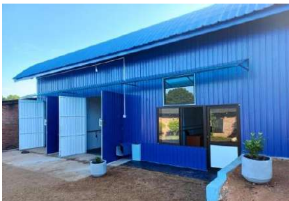
Figure 8-6: New painting facility at Halpathota
