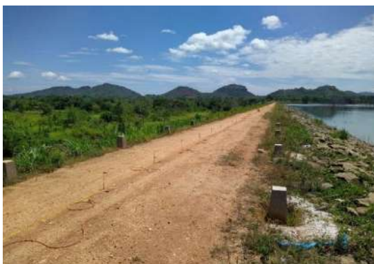
Figure 4-32: Resistivity surveying at Waththedara Morana
