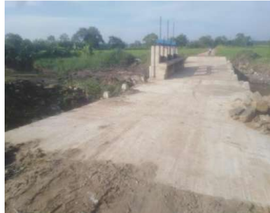
Figure 6-30: Construction of 3 bay regulators across the Woulbokkuwa drainage canal in Kaudulla
