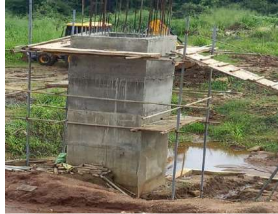
Figure 5-51: Construction of LB Sluice
