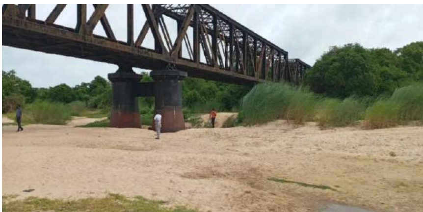
Figure 4-37: Deduru Oya river section under the Railway Bridge
