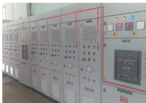
Figure 7-21: Fixing panel boards
