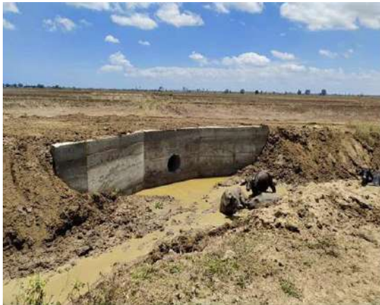
Figure 6-36: Reconstruction of off-take in Ottayanmadu bund in Sengappadai LB unit
