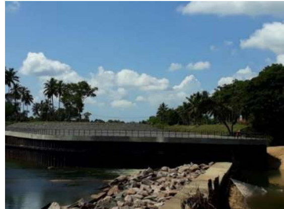
Figure 5-2: Sengal Oya sheet pile construction
