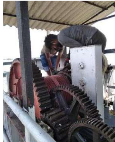
Figure 8-17: Replacing of Radial gate cables in Inginimitiya
