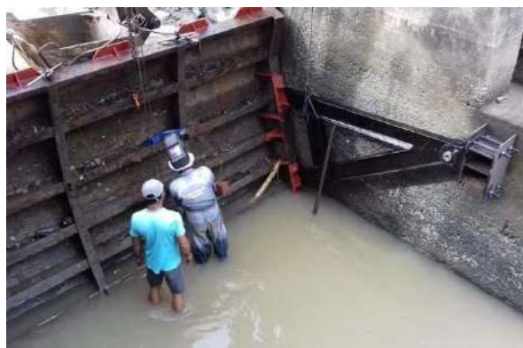
Figure 8-7: Repairing and Installation of Kirama Oya Pansala Amuna Radial Gate
