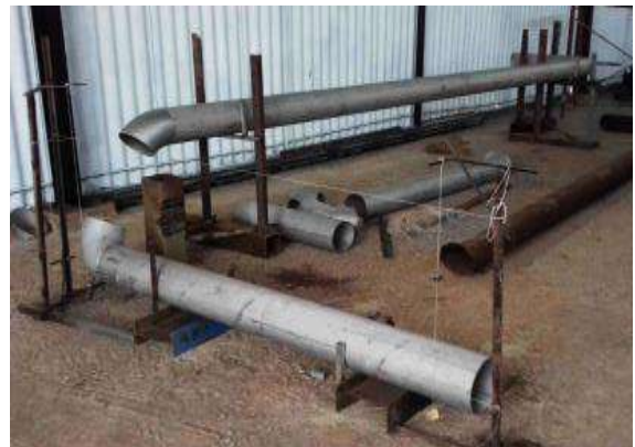
Figure 7-30: Silencer replacement Thudawa pump house
