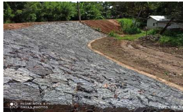
Figure 7-24: Kelani North Bund Rehabilitation
