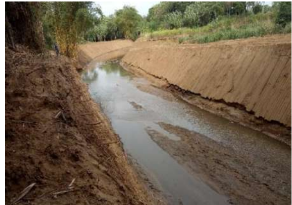
Figure 7-17: Before and after forming bund and removing formed bends along Hettipola oya
