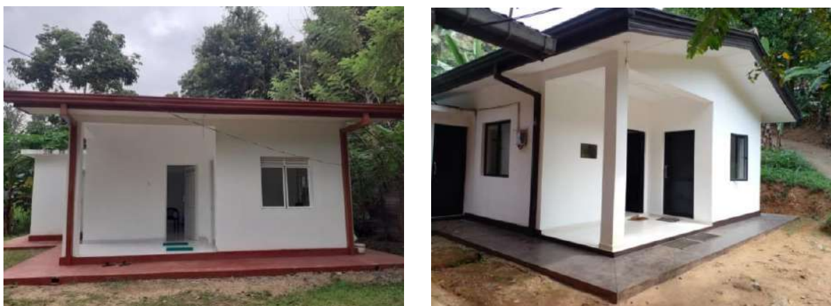
Figure 4-1: New Gauge Houses at Siyambalanduwa and Kithulgala Stations
