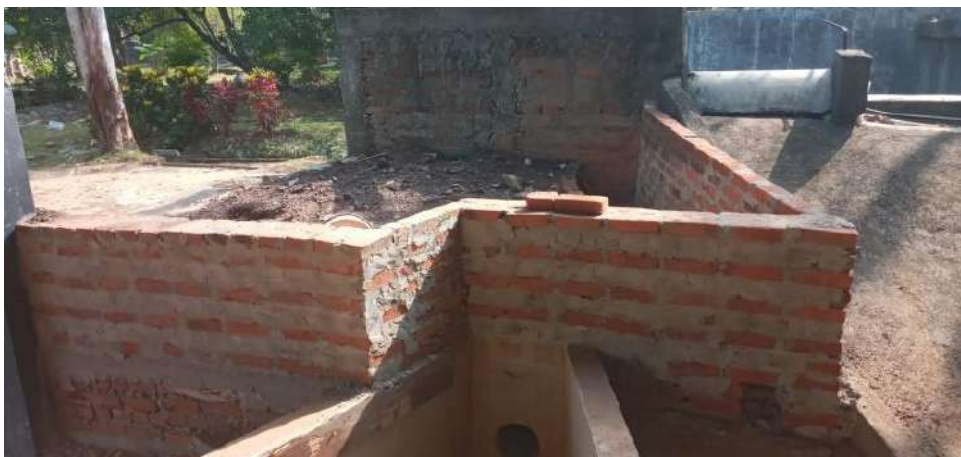
Figure 4-35: Model construction of Ellewewa uncontrolled chute spillway
