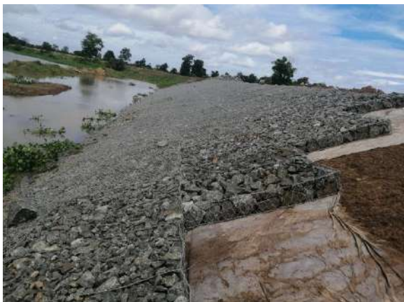
Figure 7-10: Improvements to Naathanodai Flood Protection bund from 0+270 to 0+360 in Muthur Division
