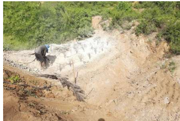
Figure 5-56: Rock Blasting work along Feeder Canal
