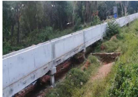
Figure 5-44: Construction of trough
