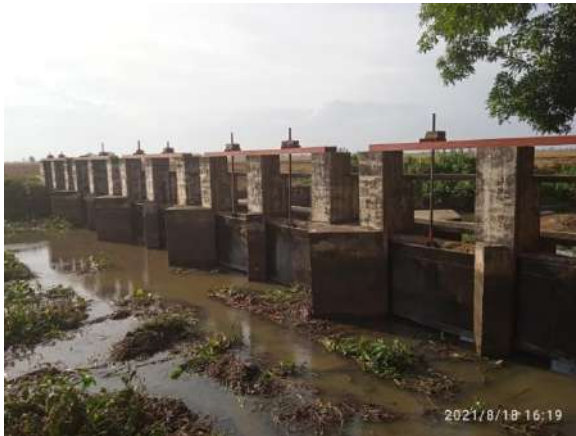
Figure 8-4: Fabrication 9Nos of New gates at Alayadiodei Annicut
