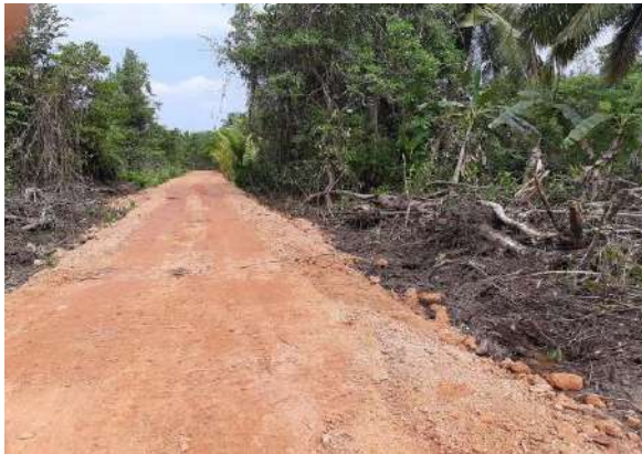
Figure 7-31: Laddauwa Warapitiya Bund construction - Bentara
