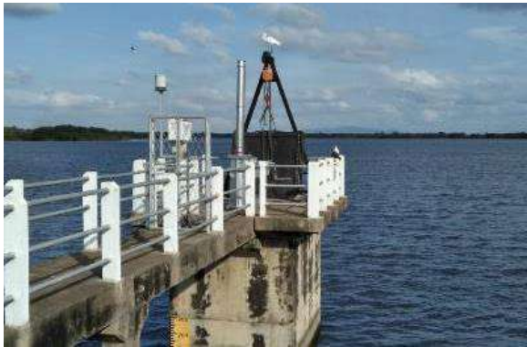
Figure 8-15: Repair of Inginimitiya RB sluice gate gear box
