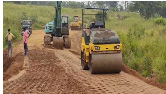
Figure 5-53: Construction of access road
