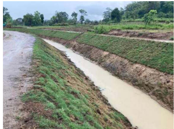
Figure 5-9: Main Canal at 10th Km
