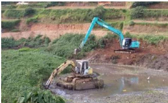
Figure 5-59: Removing Invasive plant and silt inside tank bed and supply canal
