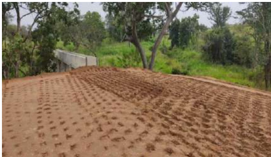
Figure 5-52: Construction of main canal
