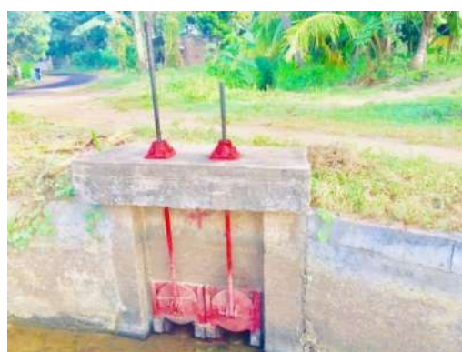
Figure 6-11: Fixing turnout gates, Kimbulwanaoaya, Kurunagala
