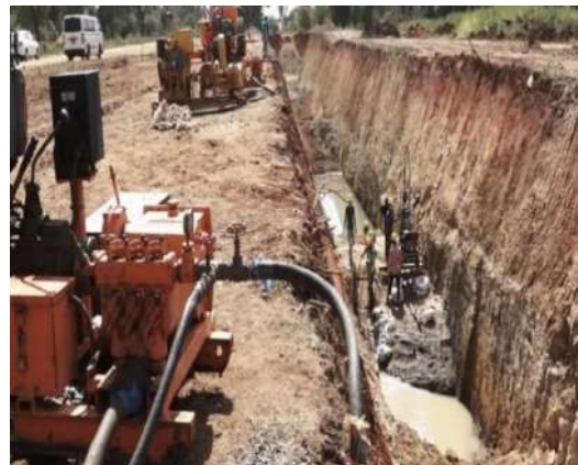
Figure 5-36: Grouting work
