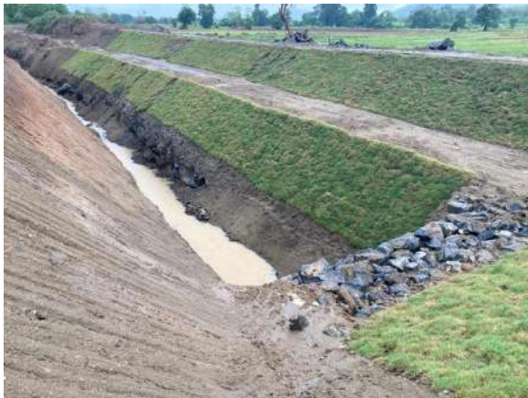
Figure 5-8: Main canal with Deep cut section at 14 km
