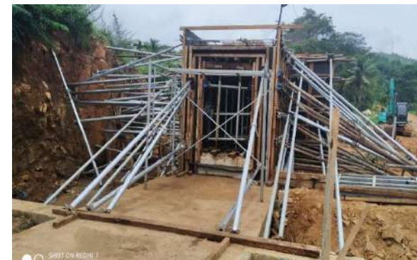
Figure 5-29 Sluice Construction
