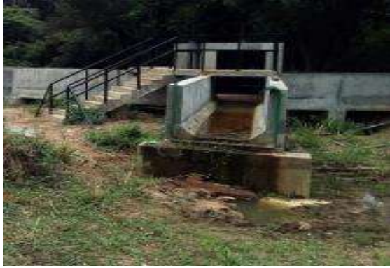
Figure 5-46: Bifurcation Structure at 0+000 and lined canal from 0+013 to 0+153 in RB canal
