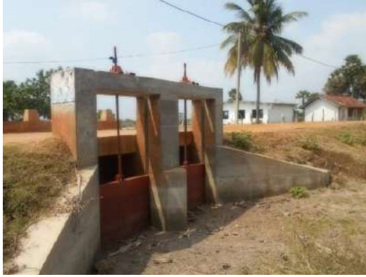
Figure 6-27: Rehabilitation of Sundikuli Feeder Tank
