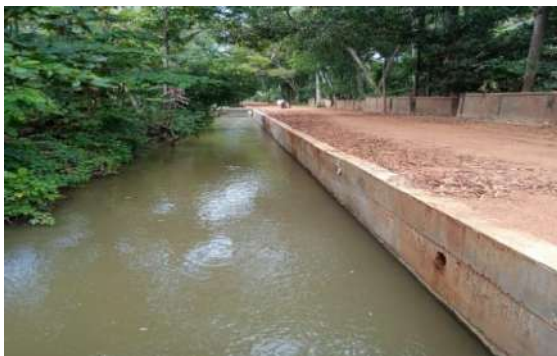
Figure 5-41: Construction of retaining wall at 1+000 to 1+333 of HLMC in Thissa Wewa
