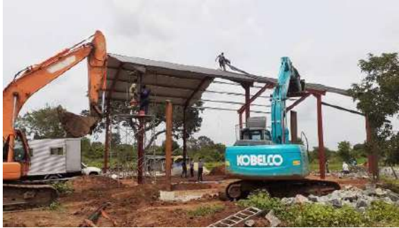
Figure 8-13: Fabrication and Erection of Malwathu Oya Workshop Building
