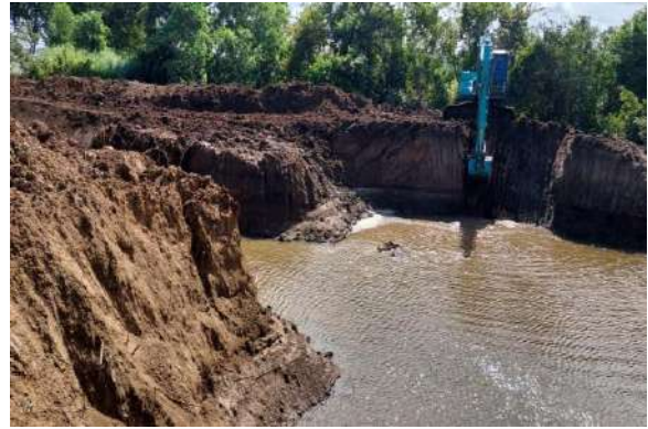
Figure 7-3: Improvements to spill tail canal from 15+550 to 16+000 in Kantale division
