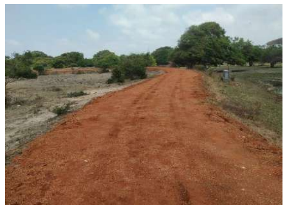
Figure 6-35: Gravelling to Maraikavoor tank bund from 0+300 to 0+600 in Akathimurippu scheme
