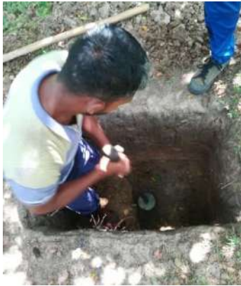
Figure 4-8: Borrow Area Investigation in Helawa Reservoir
