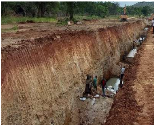
Figure 5-35: Core Trench Excavation
