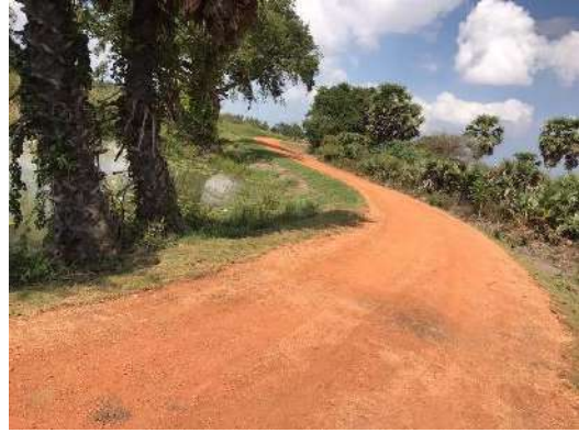
Figure 6-28: Rehabilitation of Kannaputhukulam Tank
