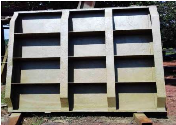
Figure 7-27: Thudawa Gravity Outlet Repair (Sand blasting & painting of Gates (06 Nos)
