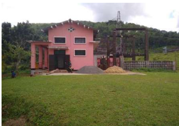
Figure 7-20: Akuretiya Pump House
