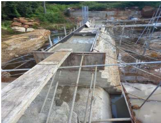
Figure 5-48: Anicut construction
