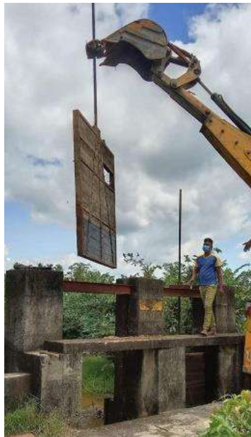
Figure 8-10: Fabrication and Installation of OU2 and Lunumadawella Gates
