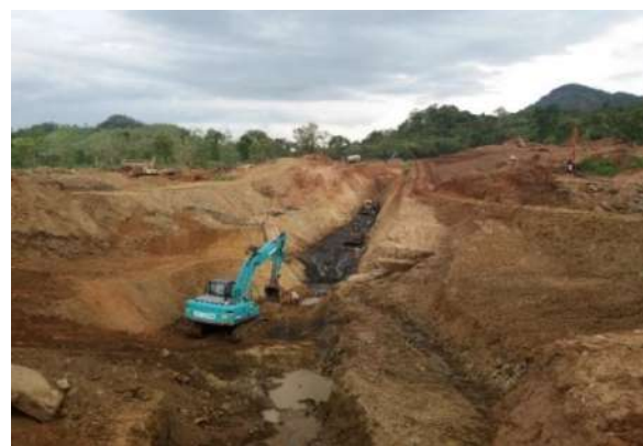
Figure 5-31 Raising of Himbilyakada Tank
