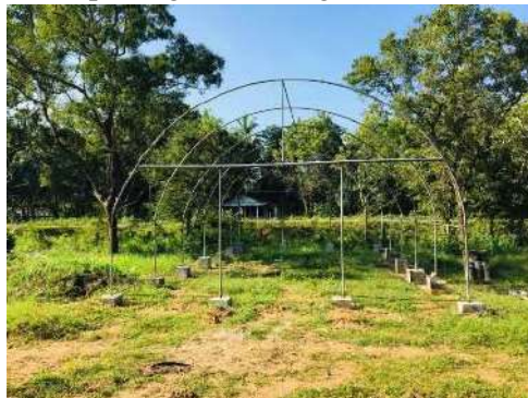
Figure 8-18: Fabrication of Green House at Kaudulla DIE's office
