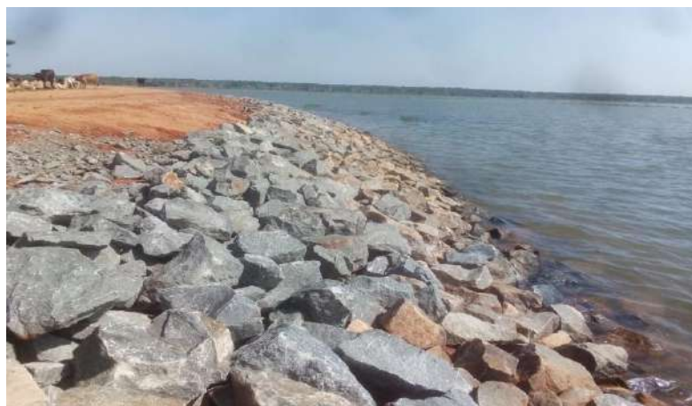
Figure 6-42: Improvements to Viyadikulam tank bund from 2+360 to 2+510 of Viyadikulam scheme
