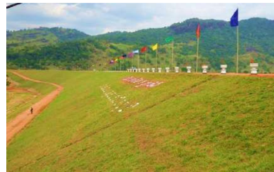
Figure 5-4: Dam of the Rambukkan Oya reservoir
