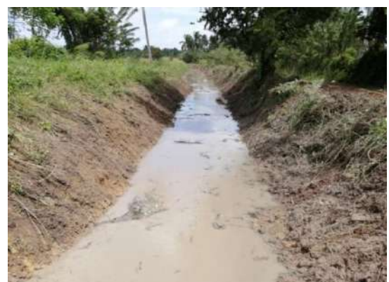
Figure 7-12: Removing invasive plants & obstacles of drainage stream at Hettirippuwa 800-1900m in Makandura
