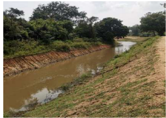
Figure 6-41: Widening of Neluoya feeder canal- Stage II in Morawewa scheme
