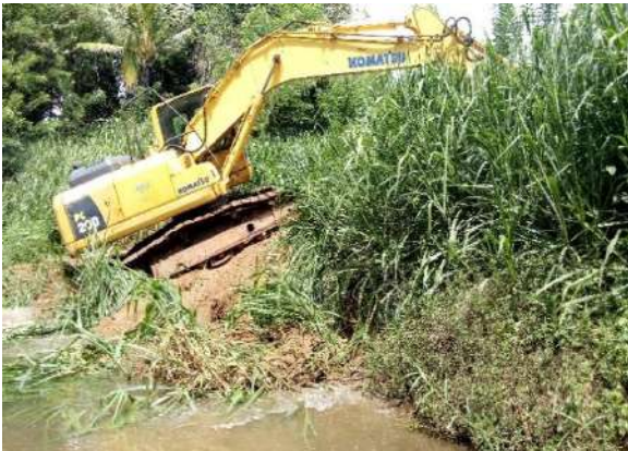
Figure 7-17: Before and after forming bund and removing formed bends along Hettipola oya
