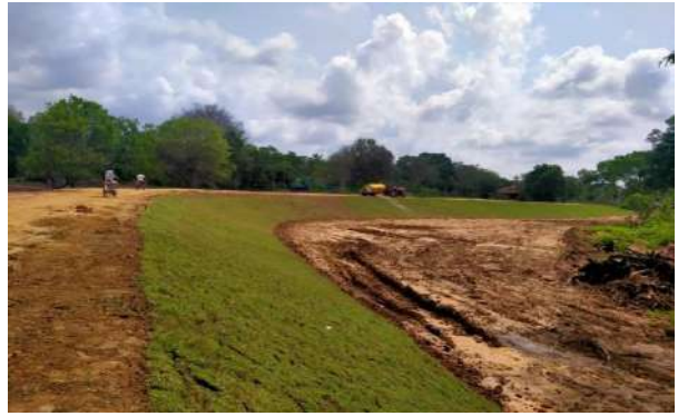
Figure 6-32: Bund Improvement in Uguressawewa, Kurunegala
