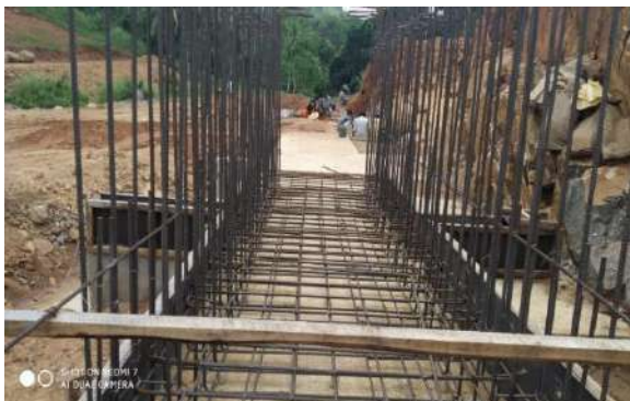
Figure 5-29 Sluice Construction
