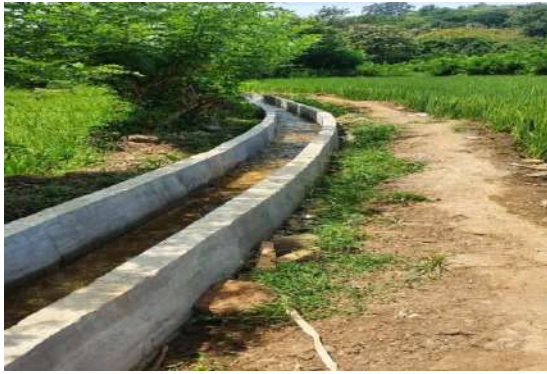
Figure 6-31: Construction of Canal in Pathagama Tank
