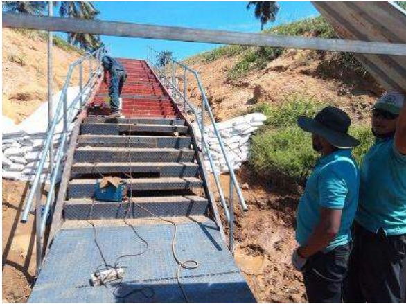
Figure 8-2: Fabrication of steel ladder and roof for "Upasampadha Pinkama" at Kaduwela
