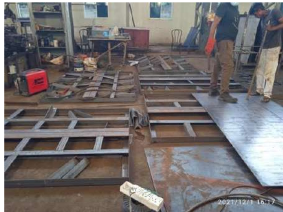
Figure 8-5: Fabrication 6Nos of New gates at Sellawali Annicut
