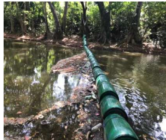
Figure 7-11: Establishment of 100m long floating trash strainer at Menik Ganga river 1st Bridge Katharagama
