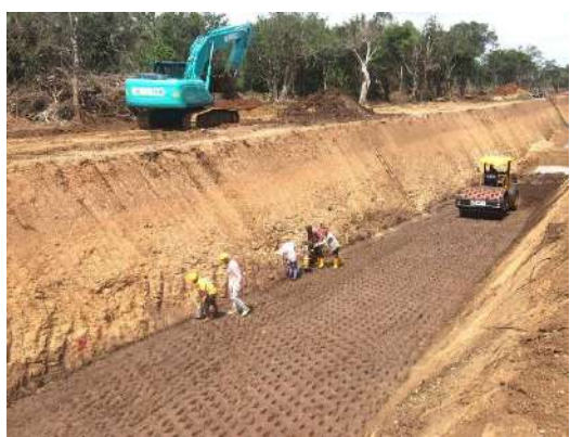
Figure 5-38: Core Trench Filling
