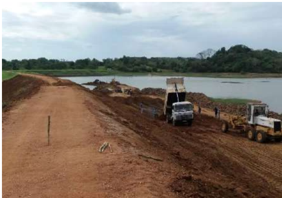
Figure 5-30 Construction of Waththegedara Tank
