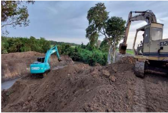
Figure 7-3: Improvements to spill tail canal from 15+550 to 16+000 in Kantale division
