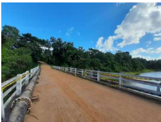
Figure 8-11: Fabrication and Installation of Muruthawela Tank Spill way Handrail
