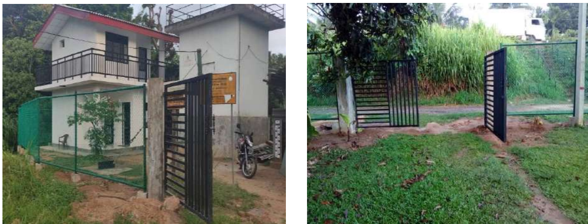
Figure 4-2: New Security Fences and Gates at Badalgama and Giriulla Stations
