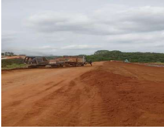
Figure 5-50: Tank Bund construction
