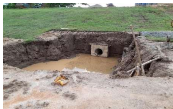
Figure 5-7: Construction of Issan Wewa Sluice
