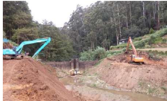
Figure 5-59: Removing Invasive plant and silt inside tank bed and supply canal
