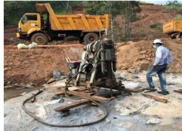
Figure 5-28: Grouting Work
