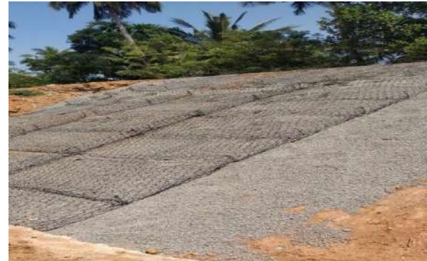
Figure 7-26: Improvements to Kelani North bund from 2+540 to 2+915
