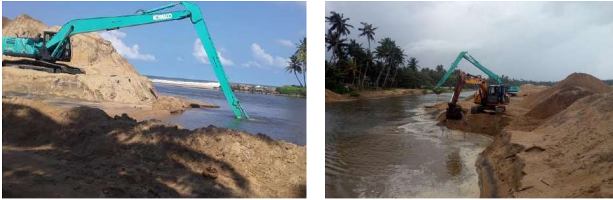
Figure 7-6: Correct the water path of Gin ganga River at River mouth Ginthota
