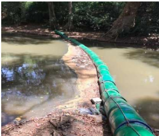
Figure 7-11: Establishment of 100m long floating trash strainer at Menik Ganga river 1st Bridge Katharagama
