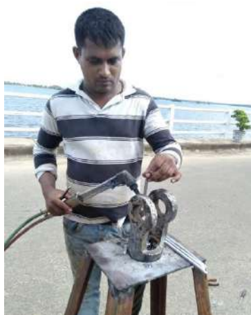
Figure 8-17: Replacing of Radial gate cables in Inginimitiya
