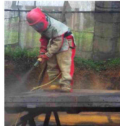
Figure 7-27: Thudawa Gravity Outlet Repair (Sand blasting & painting of Gates (06 Nos)
