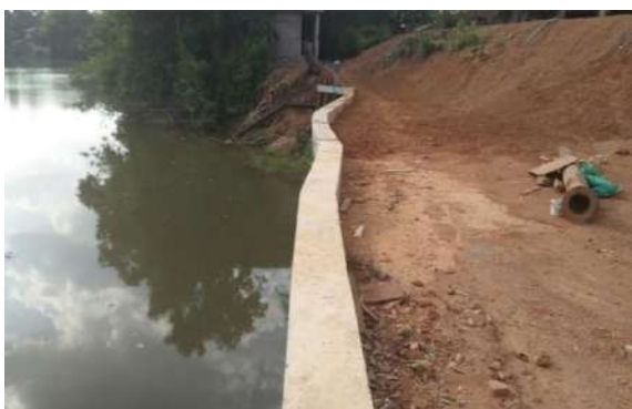
Figure 7-25: Riverbank Protection (sheet piling work)
