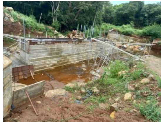
Figure 5-49: Spill way construction
