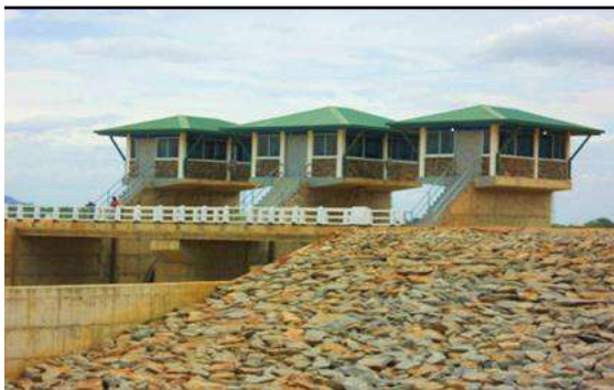
Figure 5-3: Spillway structure of the reservoir
