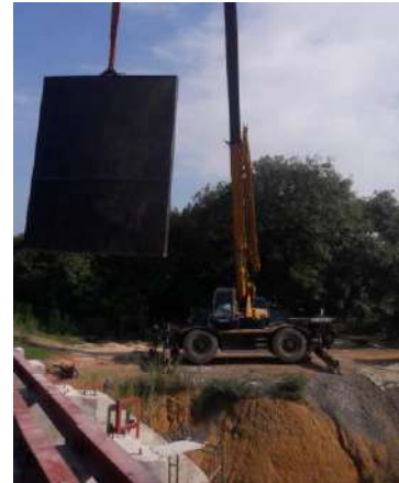
Figure 8-3: Fabrication and Installation 5Nos of new gates at Bomiriya Annicut, Kaduwela
