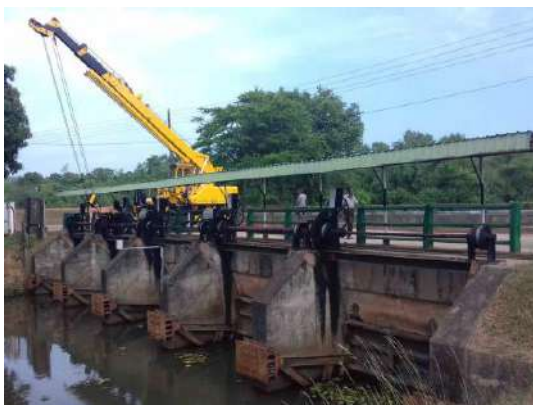
Figure 7-29: Cable Replacement of Magallagoda Radial Gate
