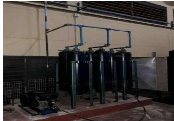
Figure 7-28: Modification of Compress Air System
