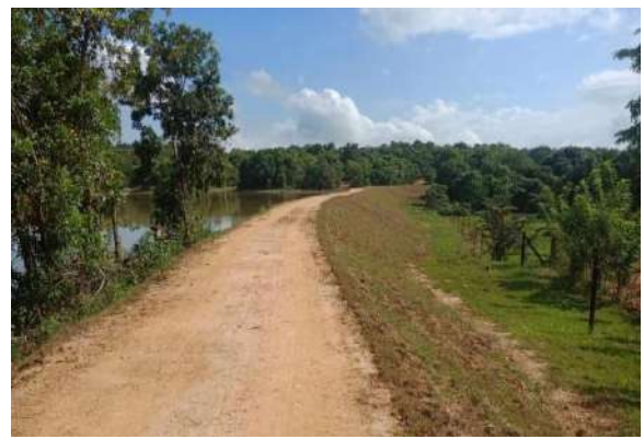
Figure 11-5: Rehabilitation of Nuwaragalathenna Tank -Mahaoya Division
