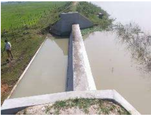
Figure 11-191: Pammanda Kulam after Rehabilitation
