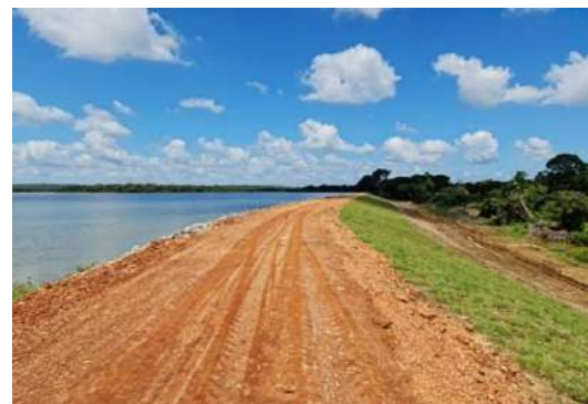
Figure 11-182: Improvements to Peramaduwa Bund
