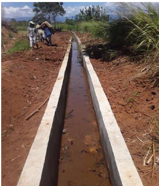
Figure 11-123: Construction of canal lining from 1+266 to 1+334 in FC17 canal - Hambegamuwa
