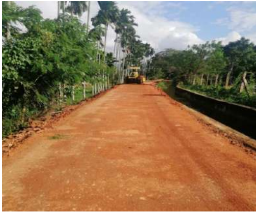
Figure 11-133: Improvements to main canal bund in Yudaganawa scheme
