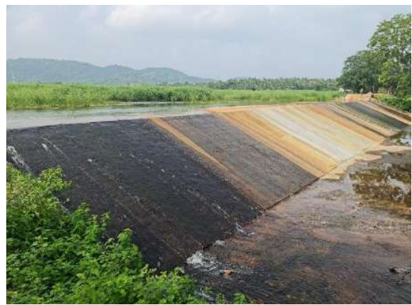
Figure 11-192: 16 Wewa after Rehabilitation
