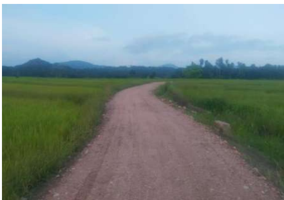
Figure 11-131: Gravelling along Thalvila canal bund road Kumbukkana scheme
