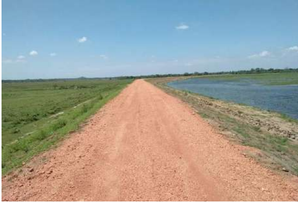
Figure 11-189: SooriyaWewa after Rehabilitation
