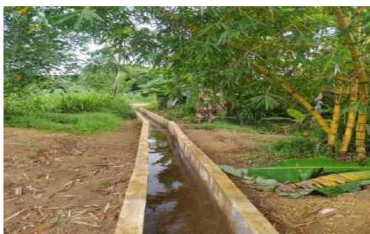
Figure 11-64: Construction of D canal in Batugedara Scheme
