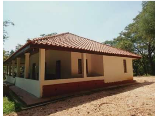
Figure 11-166: Renovation to IDEQ 01 in Elahera division
