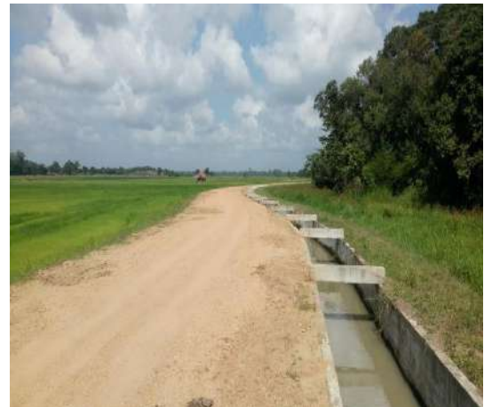
Figure 11-11: Improvement to LB cannel at Stn 0+870 to 0+960, Radella scheme
