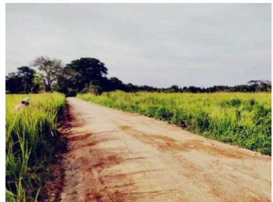
Figure 11-132: Gravelling of DC1 bund road in Ethimale scheme
