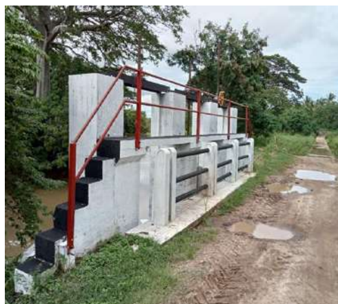
Figure 11-161 : Construction of Pinamankada Anicut in Minneriya Division
