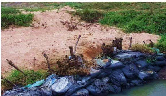
Figure 11-39: Temporary Sand Dam
