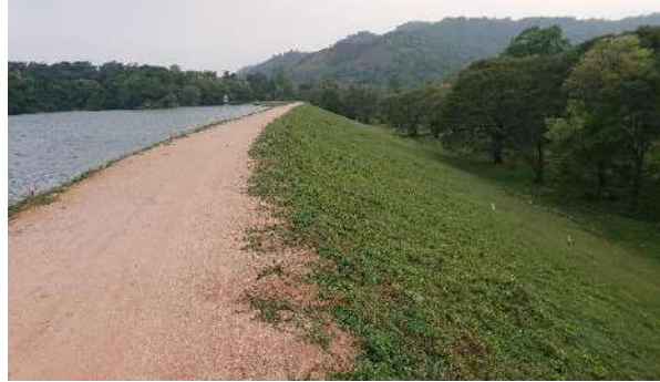
Figure 11-23: Gravelling along the bund road in Mapakada scheme
