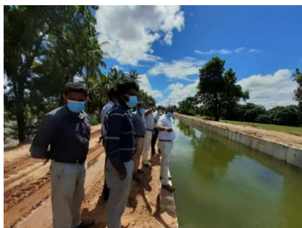
Figure 11-150: Construction of D1 North canal lining in PSS
