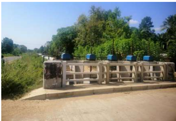
Figure 11-154: Construction of Bifurcation Structure in Damsopura Project
