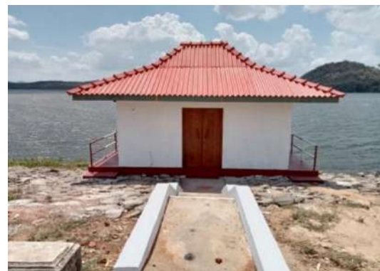
Figure 11-168: Construction of Sluice House for Girithale Tank
