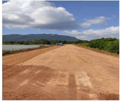
Figure 11-134: Earth filling and gravelling tank bund road Saddhathissa wewa
