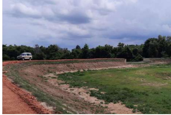
Figure 11-190: Viharagala Tank after Rehabilitation
