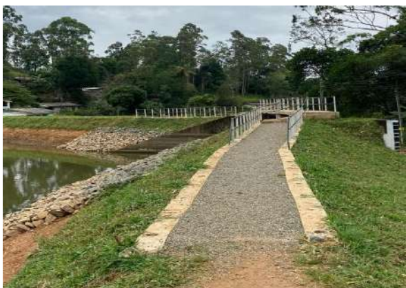
Figure 11-26- Construction of Canal lining at 4+400 at Mathotilla scheme
