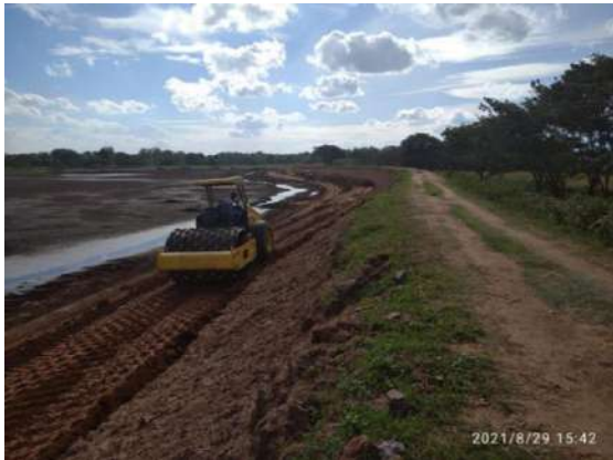
Figure 11-162: Construction of Bebiya Wewa in Kaudulla Division
