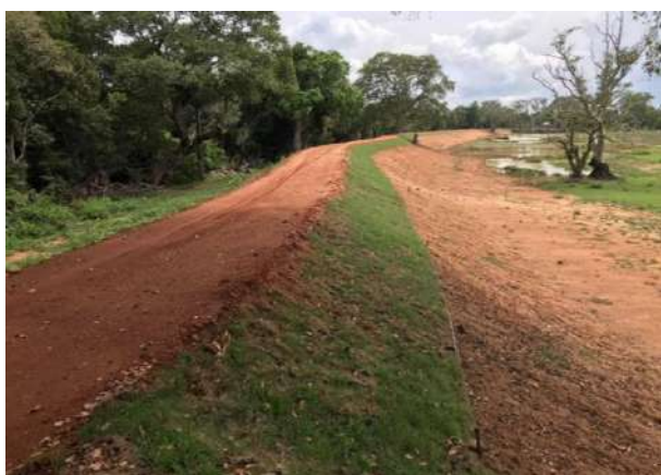
Figure 11-160: Construction of Meegas Wewa in Kaudulla Division
