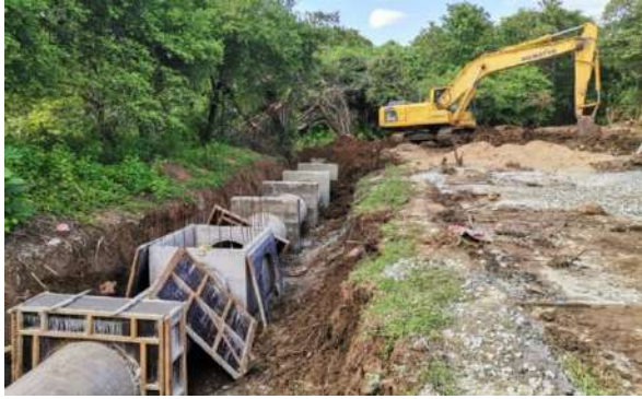
Figure 11-152: Construction of Hume pipelining in Heeratioya main canal in Heeratioya scheme
