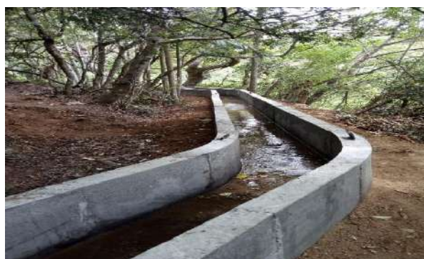
Figure 11-97: Thune Kotuwa Canal
