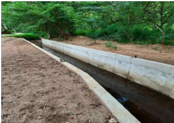
Figure 11-24-Construction of canal lining at 8+472 km in Komarika ela scheme
