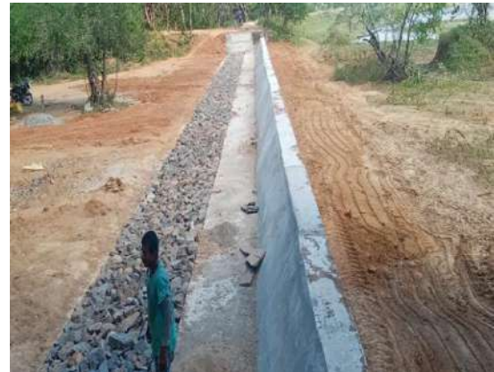
Figure 11-163: Rehabilitation of Palu Wewa in Minneriya Division
