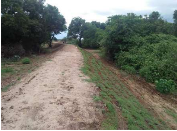
Figure 11-183: Improvements to Sooriyapura flood Protection bund
