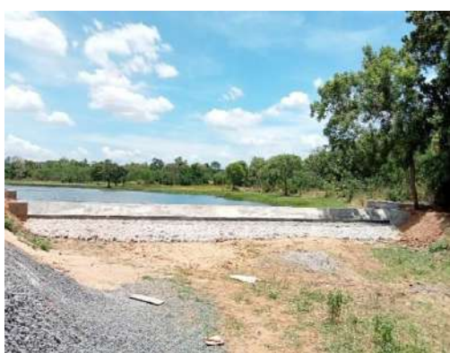
Figure 11-158: Improvements to Spillway of Kiritipitiya Tank in Minneriya
