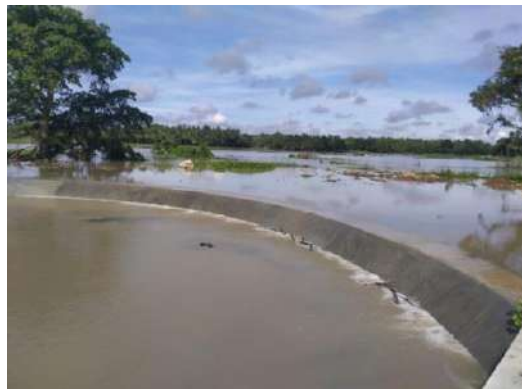
Figure 11-113: Improvements to Ambogama spill
