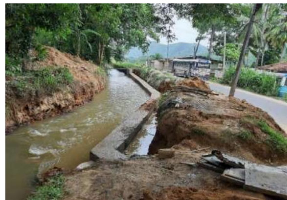
Figure 11-25-Construction 32m long retaining walla at1+488 in LBMC Bathmedilla Scheme
