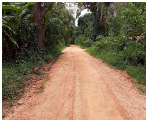
Figure 11-157: Gravelling of Girithale Main canal bund road from 0+850 to 3+250 in Girithale scheme
