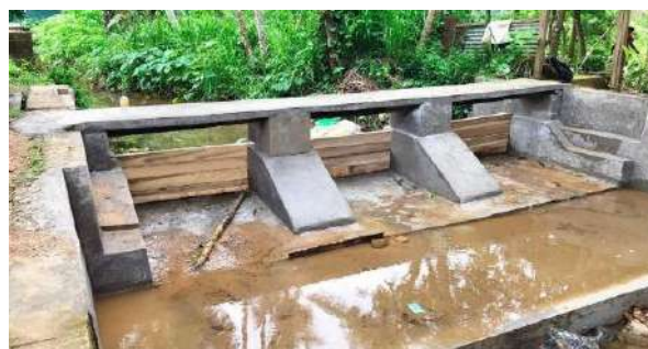
Figure 11-67: Construction Palanthiriya Anicut
