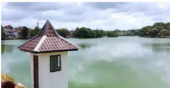
Figure 11-62: Improvements to Sluice Tower Borelasgamuwa Tank
