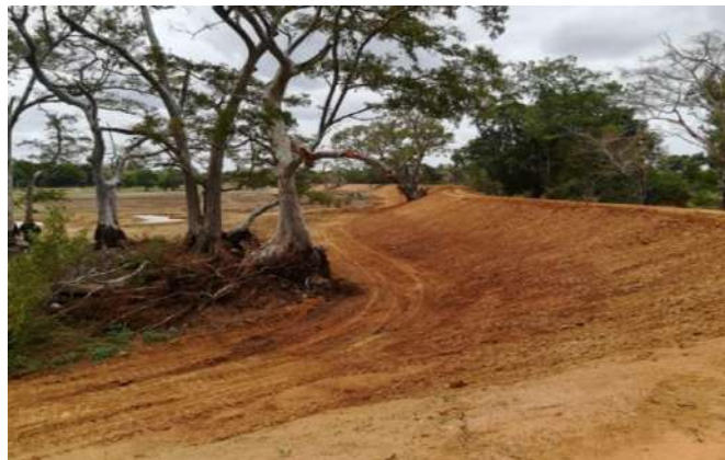
Figure 11-164: Rehabilitation of Madyamala Wewa in Minneriya Division
