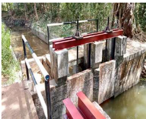
Figure 11-156: Improvements of Thambalawewa D6 diversion structure in Girithale scheme
