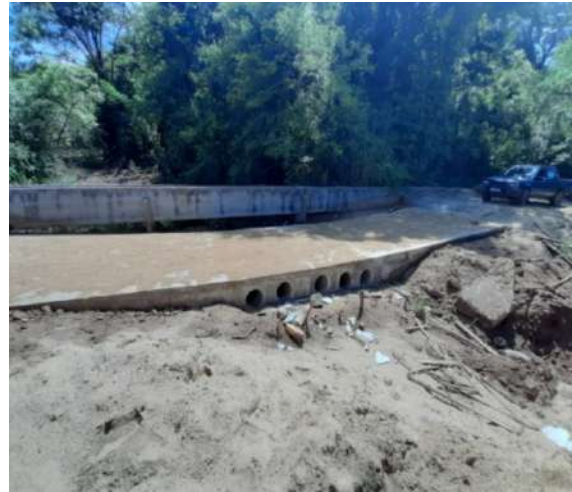
Figure 11-122: Construction of Magandanaoya main canal (5+290)
