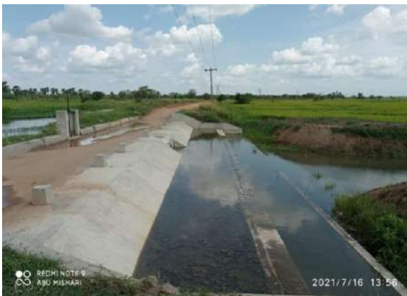
Figure 11-187: Improvements to spill no 6 in Muththur scheme
