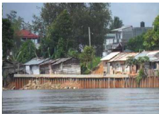
Figure 11-57: Driving Sheet piles at stage (1+678-1+718m)
