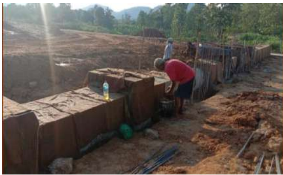
Figure 11-135: Rehabilitation of Pailegama Tank
