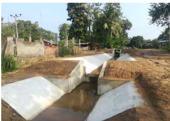
Figure 11-12: AL-10 Canal, Ambalan oya scheme
