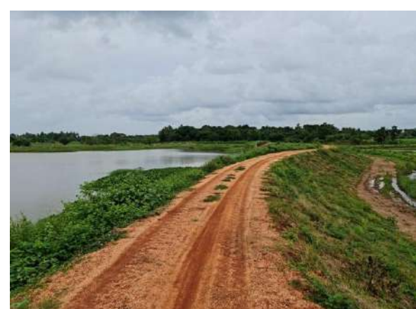
Figure 11-194: Olugollawa wewa after Rehabilitation
