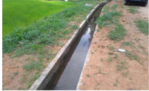
Figure 11-153: Construction of Canal lining from 0+200 to 0+300 in FC 7 in Track 33 FO area in System 'G' in Elahera Division
