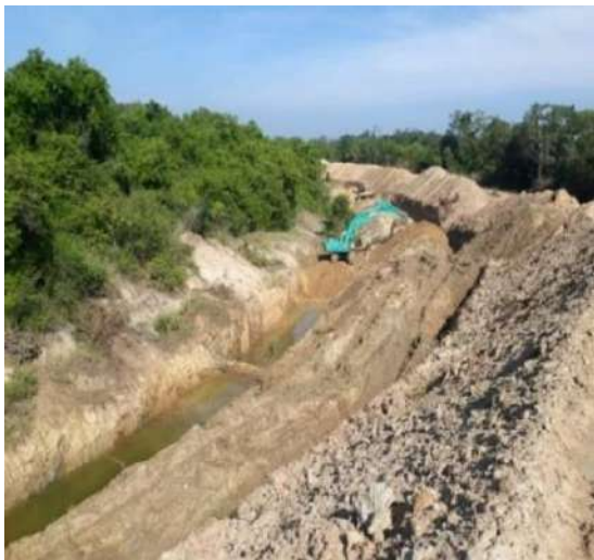
Figure 11-15: Excavation of Feeder Canal
