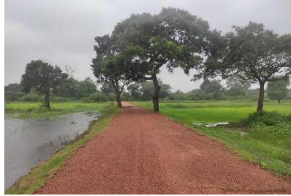
Figure 11-117: Rehabilitation of Noorganikulam
