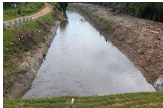
Figure 11-180: Widening of Nelu oya Feeder canal
