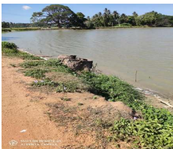
Figure 11-89: Before and after Cut Opening the Bund, Removing Roots & Refiling Debarawewa Tank Bund From 0+696 - 0+804
