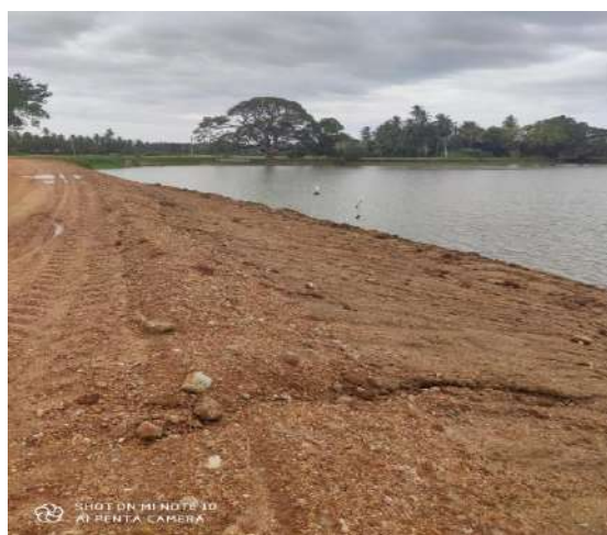
Figure 11-89: Before and after Cut Opening the Bund, Removing Roots & Refiling Debarawewa Tank Bund From 0+696 - 0+804
