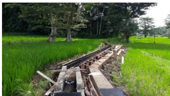
Figure 11-65: Construction Rukmale anicut
