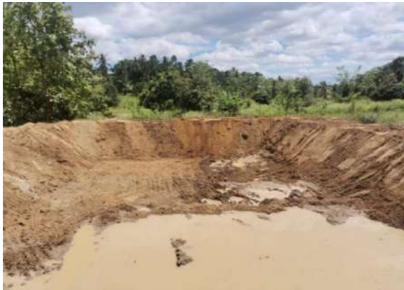
Figure 11-129: Clearing works of rainwater ponds in Dry farm Muthukandiya
