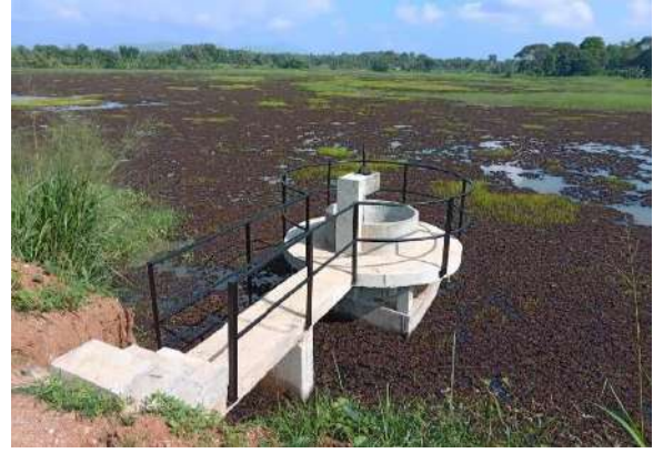
Figure 11-3: Improvements to Aaraichi Awliyada Regulator in Akkaraipattu
