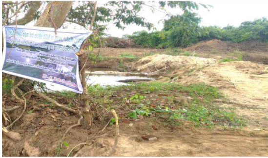
Figure 11-41: Temporary Sand Dam
