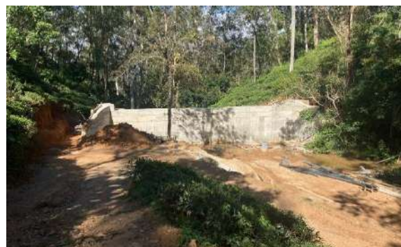
Figure 11-29- Construction of Dambagolla Tank
