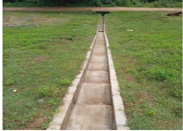
Figure 11-184: Construction of Surface drainage in kanthale Dam
