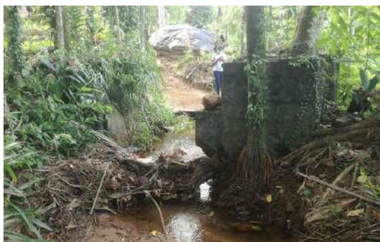
Figure 11-68: Before Construction Hopitigala Amuna, Rathnapura Division
