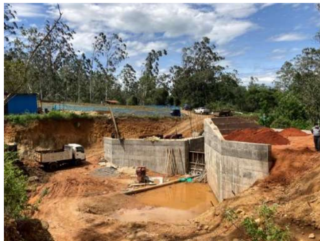
Figure 11-20: Construction of Dimbulaththa Tank
