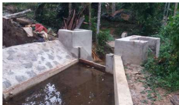
Figure 11-69: After Construction Hopitigala Amuna, Rathnapura Division
