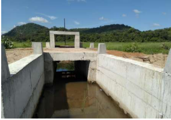
Figure 11-2: Improvements to Aaraichi Awliyada Regulator in Akkaraipattu
