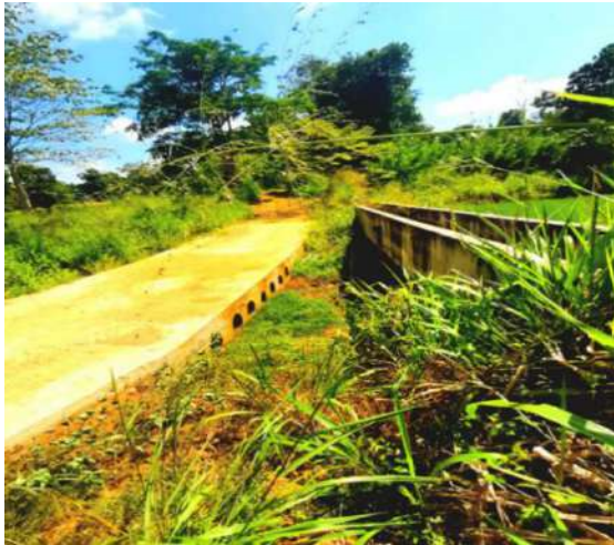
Figure 11-121: Construction of Magandanaoya D canal (5+227)
