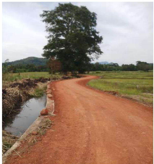
Figure 11-124: Gravelling Sudupanawela canal bund road 3+250 to 3+935
