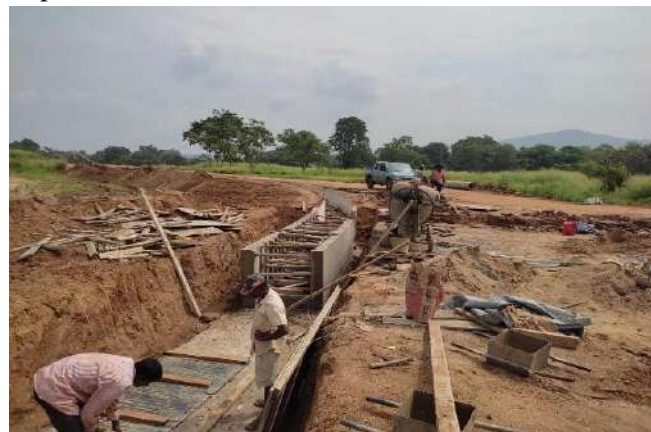
Figure 11-21: Construction of canal lining of Wilakandiya project
