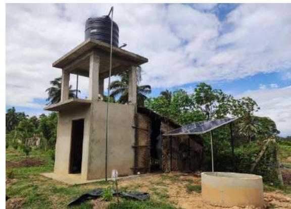
Figure 11-86: Construction of Water supply system for farm at Udukiriwila model farm
