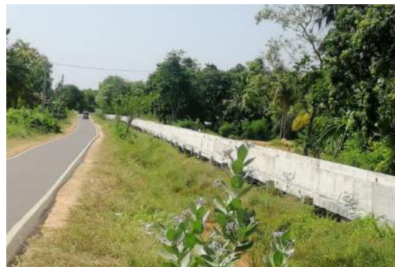
Figure 11-155: Construction of Trough in Damsopura Project II
