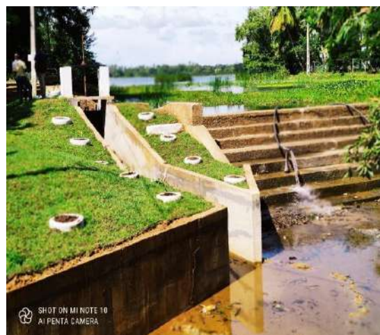
Figure 11-88: Before and after construction of new spill gate at Debarawewa tank
