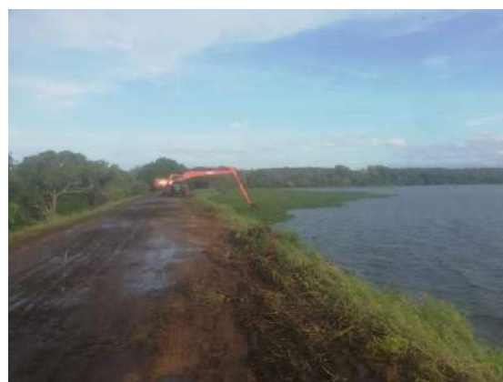
Figure 11-18: Removing aquatic plants in Galkulama tank
