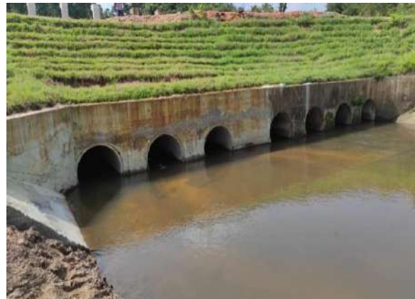
Figure 11-188: Improvements to Neluoya Inlet structure
