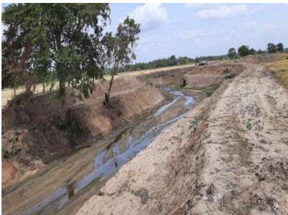
Figure 11-185: Improvements to Kanthale spill tail canal
