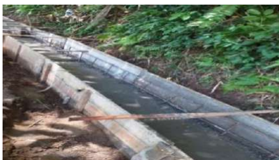
Figure 11-66: Construction Pothuwil anicut and main canal
