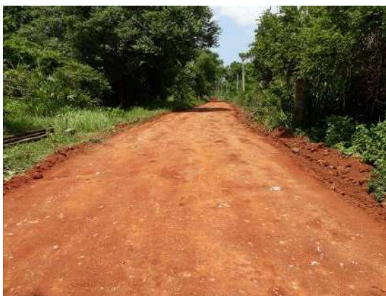
Figure 11-17: D11 UMC road after construction
