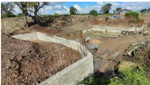
Figure 11-181: Construction of Pan oya Anicut
