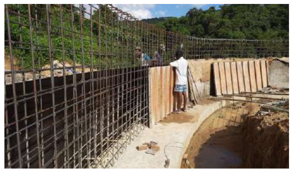
Figure 11-136: Rehabilitation of Moragolla Tank
