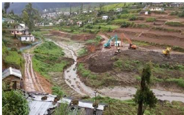
Figure 11-92: Desilting work at Barrack plane tank
