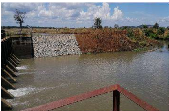
Figure 11-178: Improvements to D/S of the Pirambuveli Anicut in Raja Ela Canal at stn 14+200 in Allai Extension Scheme in Muthur Division
