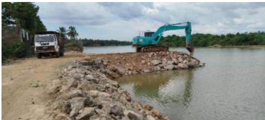
Figure 11-170: Construction of Groyne 02 (Stage 2) in Jayabima Area in Deduru Oya
