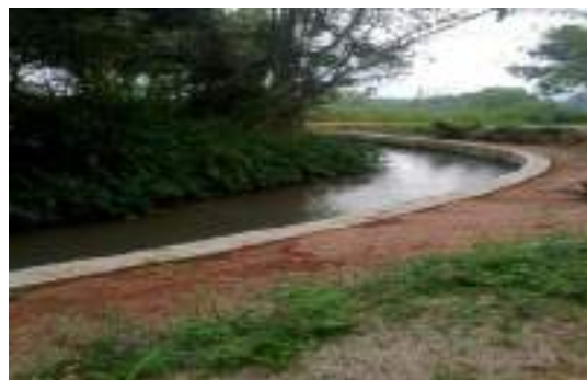
Figure 11-159: Construction of 60 m long retaining wall structure from stn.3+100 to stn.3+160 in Nikapitiya D canal
