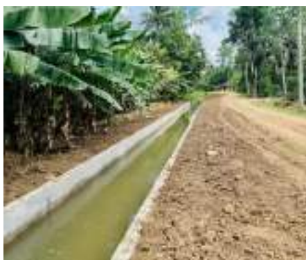
Figure 6-20: Improvements to FC 54 canal in track II in Muruthawela scheme in Hambanthota Region
