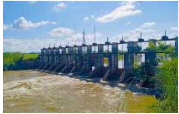
Figure 11-70: Supplying and installing steel gate with component to Kochcharasenai anicut in Unnichchai
