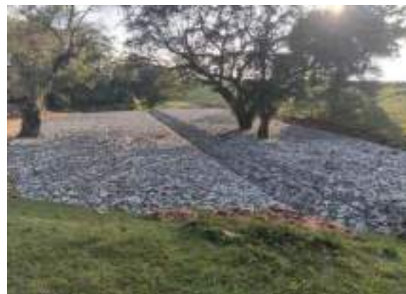
Figure 6-17: Providing loading berm at PSS
