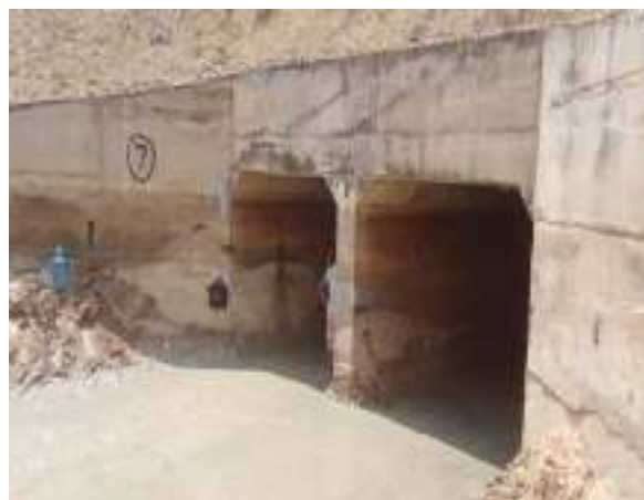
Figure 11-172: Clearing aquatic plants and desilting along Deduru Oya RBMC from 30+000km to 36+700km in Inginimitiya Division
