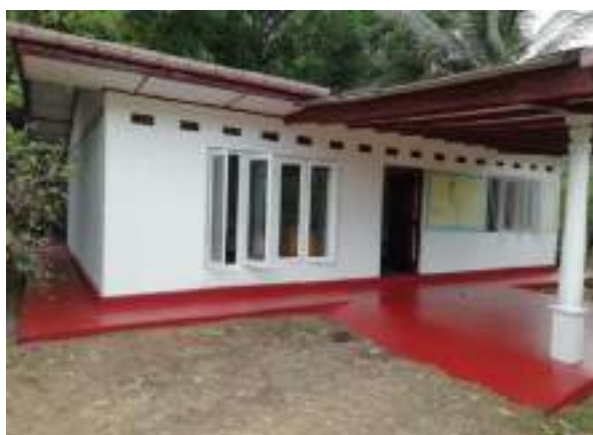
Figure 11-41: Repairs to Unit Office at Thaldena Scheme. / Unit Office
