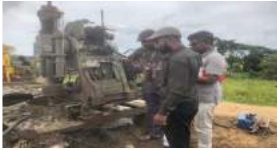
Figure 4-9: Treatment for a Leakage through Weeravila Tank Bund in Thissamaharama Division
