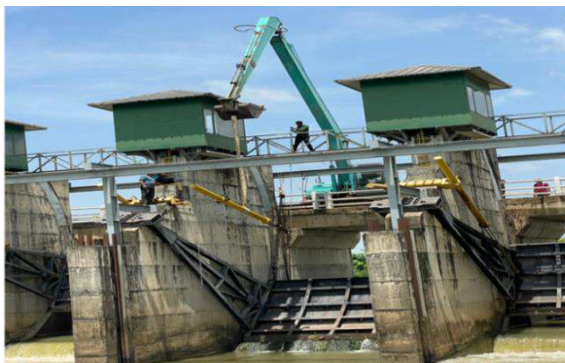
Figure 11-57: Service and repair to Mavadiodai anicut gates in Rugam Division
