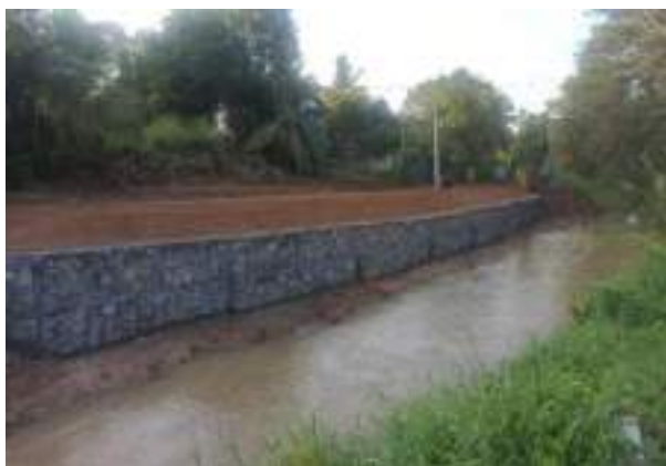
Figure 7-6: Construction of protection wall for kirama oya RB side at downstream of Danketiya anicut in Kirama oya scheme in Hambantota Region
