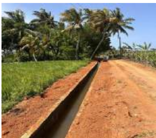
Figure 11-95: Improvements to Construction of protection wall 27 canal in SCB canal Beragama unit -WLB Scheme.
