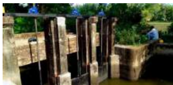
Figure 11-186: Fabrication & Installation of 03 Nos of mild steel gates with Screw type hoisting mechanisms for Wendrasan Raja Amuna Regulator in Kantale Division, Trincomalee
