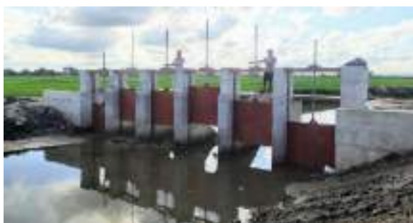
Figure 11-65: Construction of Naasivanvelly regulator in Kallathu drainage channel in Unnichchai scheme
