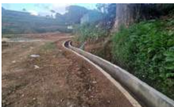
Figure 11-110: 0+000 to 0+300 side drain Construction
