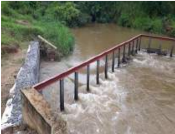
Figure 11-118: Strengthening of both up stream side of Syphon at 11+346 in Minipe LBMC
