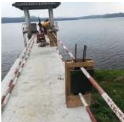
Figure 11-187: Improvements to Morawewa Reservoir Sluice
