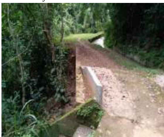
Figure 11-36: Improvements to canal spill 0+810 km in Komarika ela Scheme / WM
