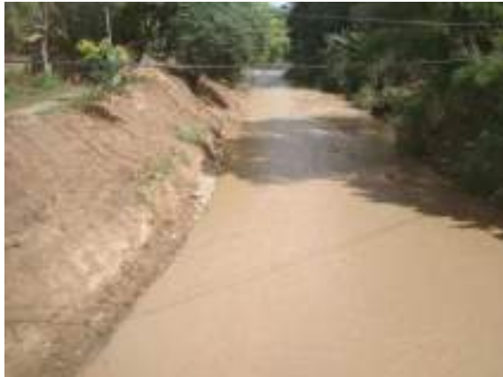
Figure 11-43: Removing silt deposits, common excavation in Deiyannewela near bridge in Badulu Oya / Establishing River Profile
