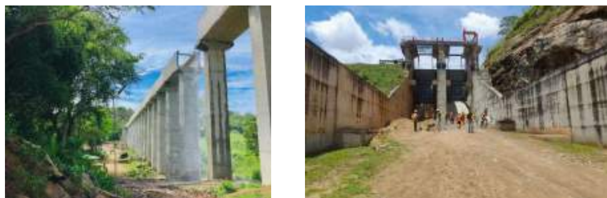
Figure 5-7: Uma Oya Downstream Development Project
