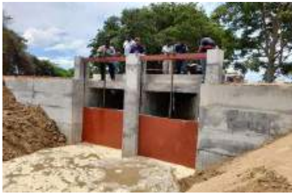
Figure 11-71: Improvements to Peelimadu Bridge cum regulator in Vahanery Scheme,
