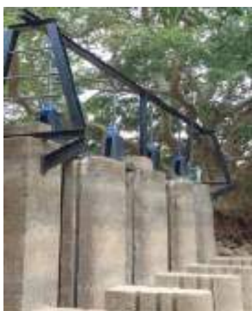
Figure 11-185: Improvements to gates & hoisting system and fabrication and Installation of Trash racks and handrail for Batahathara Regulator in Kantale Division
