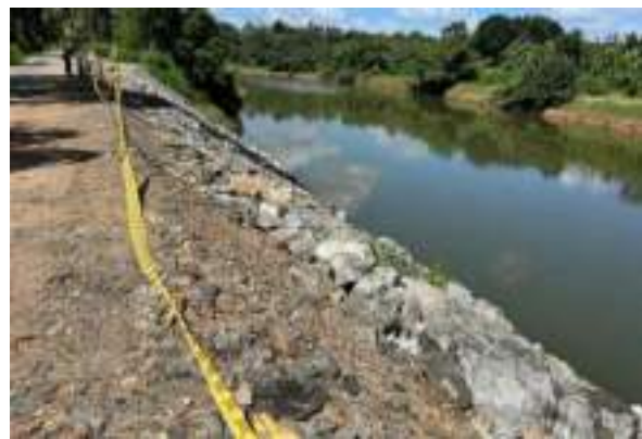
Figure 7-12: River Bank Protection (Before and after boulder packing at Akarawita)
