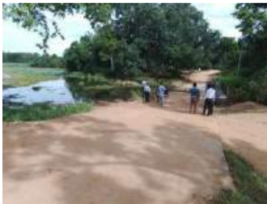
Figure 6-22: Arawatta tank bund and spill way in Mapakada Division - Badulla Region
