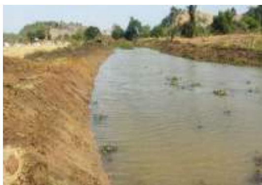
Figure 11-183: Deepening and widening drainage canal stn. 2+000 to stn. 2+910 in Santhanaveddai in Allai Extension Scheme
