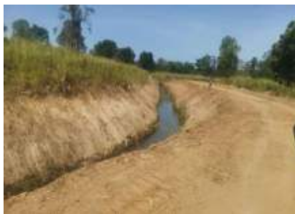
Figure 11-29: Desilting in LB Main canal 6+000km 12+000km
