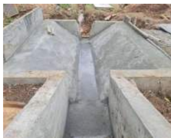
Figure 11-117: Construction of drop structures in FC-01, FC-03, FC-05 at RBMC in Mahagonawewa scheme
