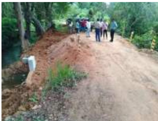
Figure 6-24: Construction progress inspection of Hanththota amuna in Mathale Division – Kandy Region
