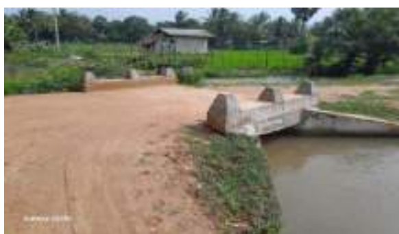
Figure 11-146: Construction of box culvert at Issaimalaithalvu canal end
