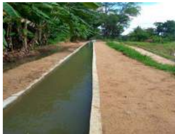
Figure 11-119: Improvements to D34 canal from 0+620 to 0+737 in stage II
