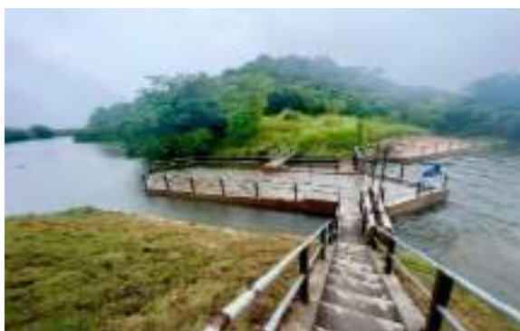
Figure 5-10: Construction of outlet structure at 0+000
