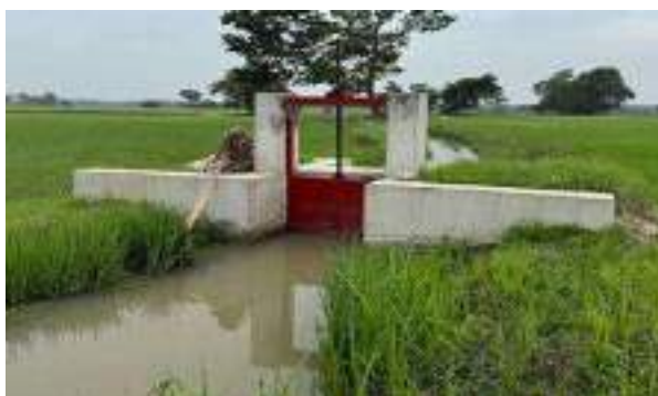
Figure 11-61: Construction of Regulators along Sanmugarajah sub supply chl. At stn 0+385,0+765 & 1+050 in Navakiri scheme
