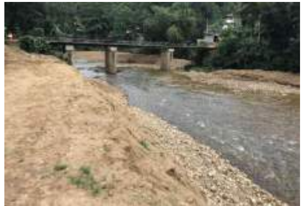
Figure 11-44: Removing silt deposits and common excavation in Ekanayaka mawatha near bridge (Egodagma) / Establishing River Profile
