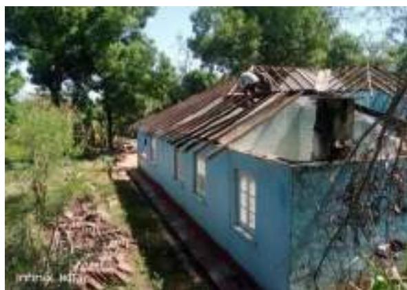
Figure 11-39: Repairs to Baduluoya Unit Office in Kandaketiya division / Unit Office
