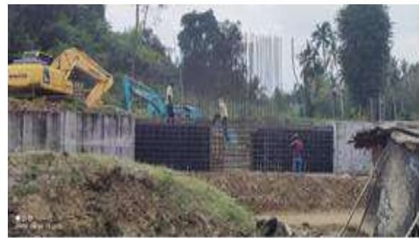
Figure 4-11: Foundation Sealing for Ellewewa Dam
