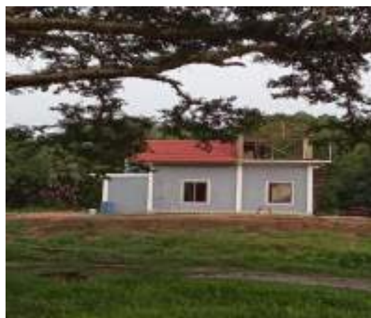
Figure 6-11: Improvements to Kithuluthuwa Unit Office in Kantale Division
