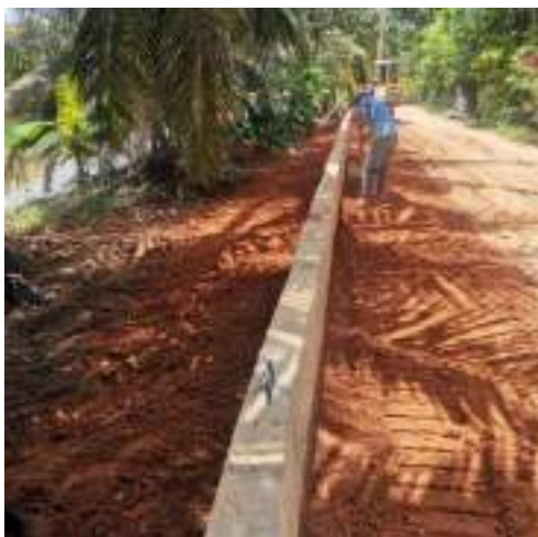
Figure 7-15: Construction of Flood Protection wall in Ja-Ela Flood bund
