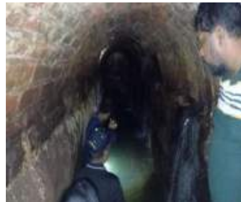
Figure 6-25: Inspection of Magalla wewa sluice.
