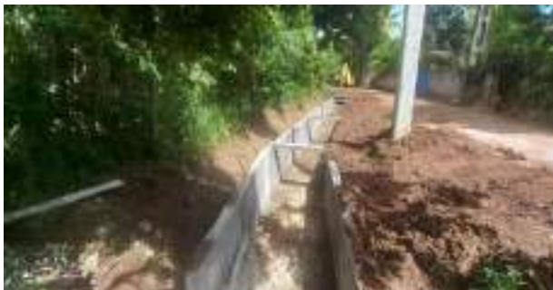
Figure 11-86: Improvements to Ellakanda main canal construction of canal lining from 2+880 to 3+030 in Kekanadura scheme
