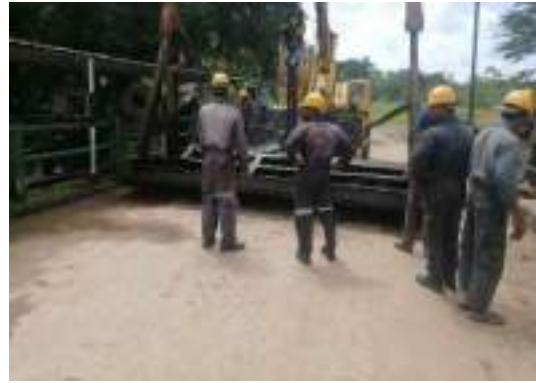
Figure 7-14: Repairs to Radial gate at Magallagoda Gravity Outlet
