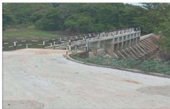
Figure 5-11: Improvements of Eru Wewa spill and tank bund RB Approach road
