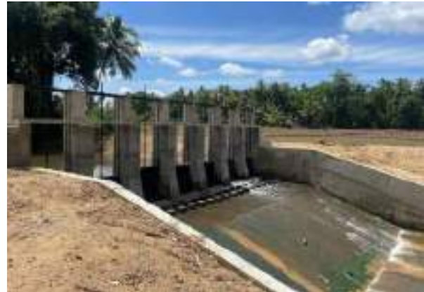
Figure 11-3: Improvement to Meegahapallama Anicut structure in Damana unit in Ampara division under CResMPA project
