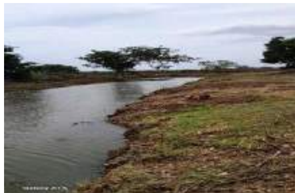
Figure 7-9: Removing water Block in Saampodai Aru Drainage Channel from 1+200 to 3+500 in Allai Extension in Muthur in Trincomalee Region
