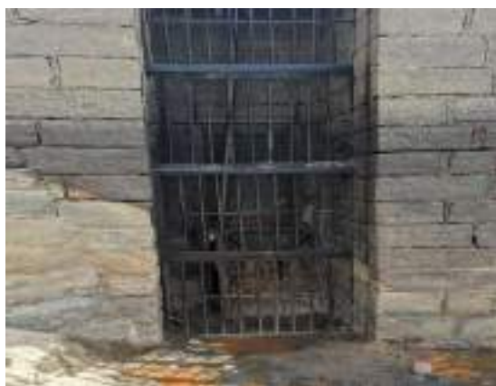
Figure 11-67: Repairs painting and installation of Vahanery tank RB sluice gate with hoisting mechanism in Rugam
