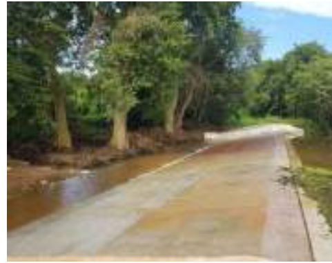
Figure 11-17: Improvements to spill at Atambagaskada tank
