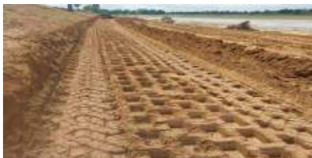
Figure 11-66: Rehabilitation of Thumpankerny tank bund from Stn, 0+000 to stn. 0+650 in Thumpankerny scheme in Navakiri Division. Batticaloa
