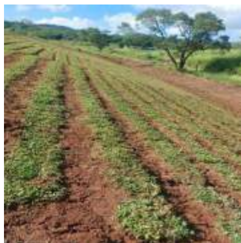
Figure 5-13: Turfing of tank bund
