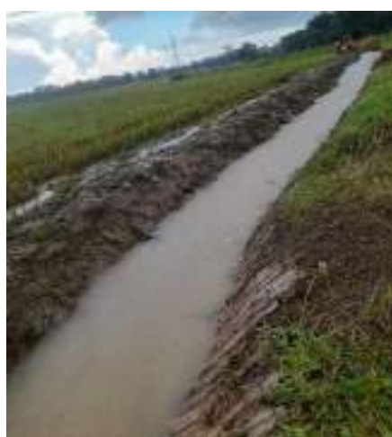
Figure 11-97: Clearing and desilting in Wile Basnawa drainage canal in Kirama oya scheme
