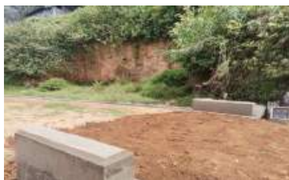
Figure 11-111: 0+080 Single pipe Culvert & Drainage
