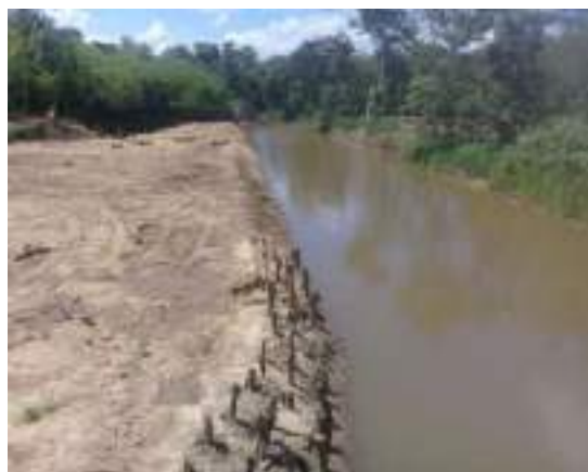
Figure 7-5: Clearing the deposited sand and protection of River Bank by constructing Gabion boxes and providing timber piles at RB embankment near Dunumewa Bridge of Gal oya in Monaragala Region
