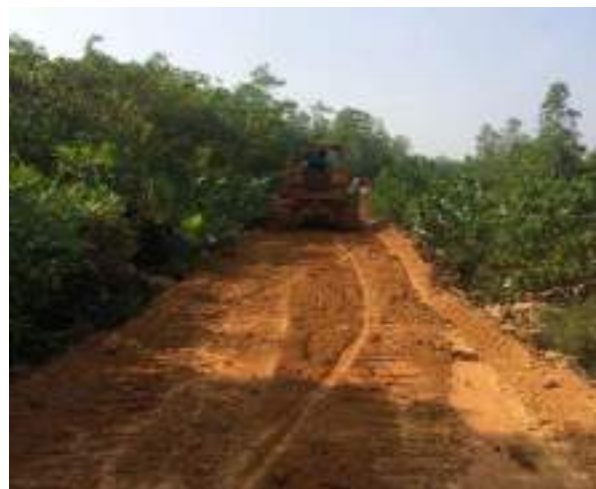
Figure 7-16: Improvements to SWE bund in Bentara LB Scheme
