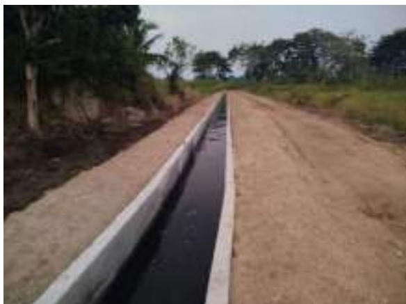
Figure 11-168: Construction of Canal Lining from 0+008.6km to 0+100km Main Canal of Kudaottupallama Tank in Neelabemma Scheme
