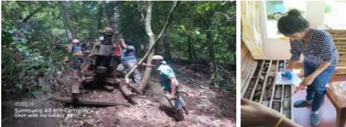
Figure 4-8: Geotechnical investigation for the proposed Wewalkandura Ara Reservoir
