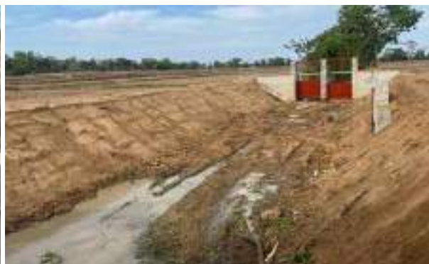
Figure 11-60: Improvement to T-9 drainage canal (Pallavaikal) in Navakiri Scheme
