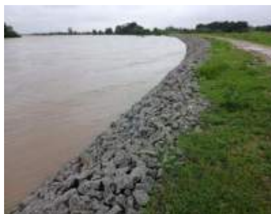
Figure 7-7: -Slop protection of Mahaweli flood protection Bund (Towards soorangal Road) from 6+800 to 7+100 in Muthur Division in Trincomalee Region
