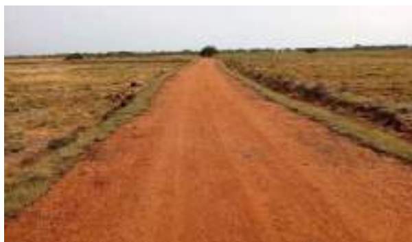
Figure 11-148: Improvements to 7 th Sluice Canal Road in Akkathimurippu Scheme
