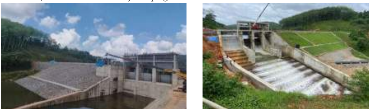
Figure 5-9: Construction of Basnagoda reservoir project
