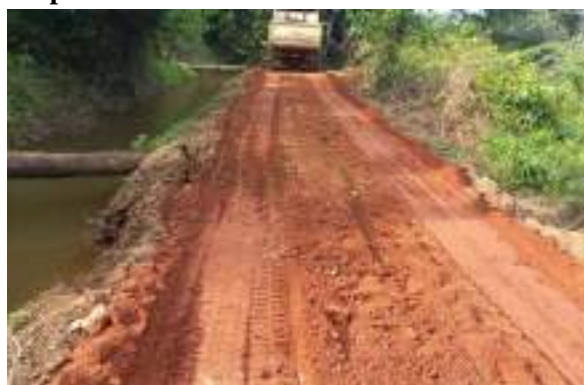
Figure 11-30: Improvements to canal bund road from 3+000 to 3+750 LBMC in Mapakada Scheme / Roads
