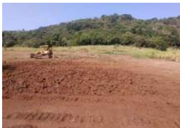
Figure 11-28: Land Levelling of Lots under D4 and D5 canal
