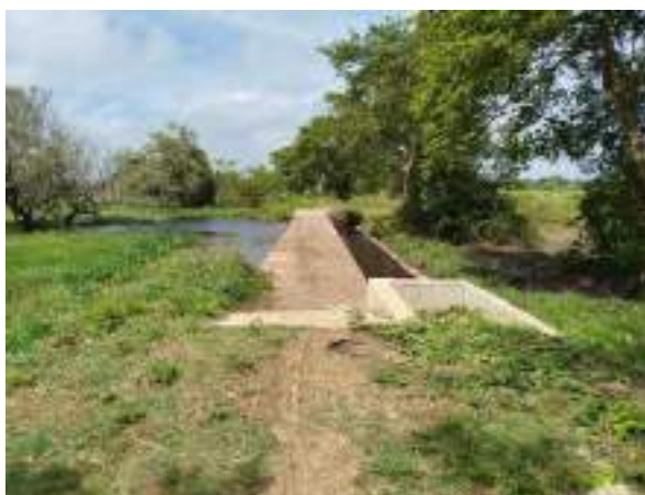
Figure 11-171: .Improvements to Spill Structure to Pinkattiya Tank in Sengal Oya Scheme
