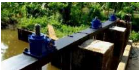
Figure 11-186: Fabrication & Installation of 03 Nos of mild steel gates with Screw type hoisting mechanisms for Wendrasan Raja Amuna Regulator in Kantale Division, Trincomalee
