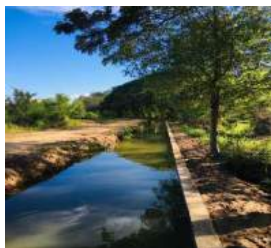
Figure 11-98: Improvements to main canal in pahala Andara Wewa.
