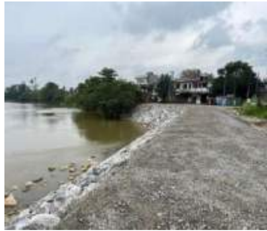
Figure 7-11: River Bank Protection (Before and after boulder packing at Kohilawaththa)
