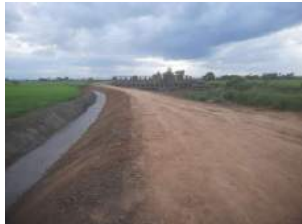
Figure 11-5: Breach filling LB & RB bunds of Moravil river in Moravil II unit in Sammanthurai division
