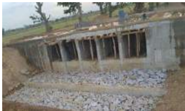
Figure 11-62: Reconstruction of Thumpalai Thikkodai connecting causeway at stn 0+404 in Navakiri scheme
