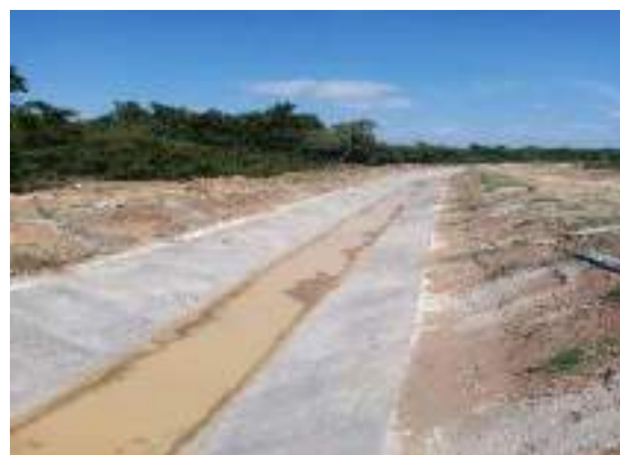
Figure 11-14: Issanwewa Main Canal
