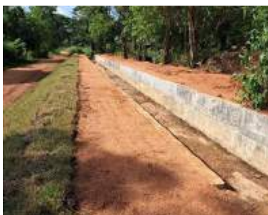
Figure 11-123: Construction of D3 canal lining at 0+700
