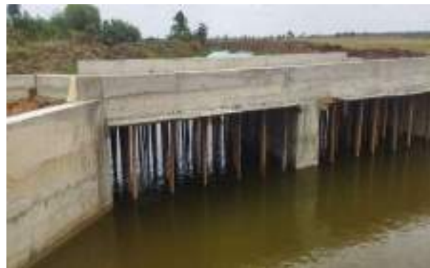
Figure 11-184: Construction of Culvert at 2+450 in Santhanaveddai Drainage Canal
