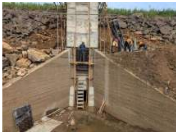
Figure 11-46: Rehabilitation of tank bund, Sluice in Nagadeepa tank.
