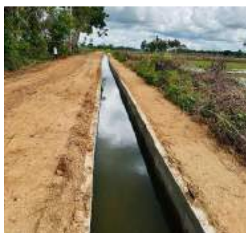
Figure 11-102: Improvements to the NCB LB 3 canal lining 0+750 to 0+990
