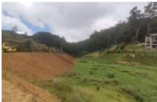
Figure 5-14: Forming approach road around the tank
