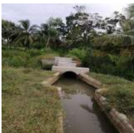
Figure 11-99: DC/208 - Improvements to RB main canal of Ranmuduwewa from 0+300 to 3+000
