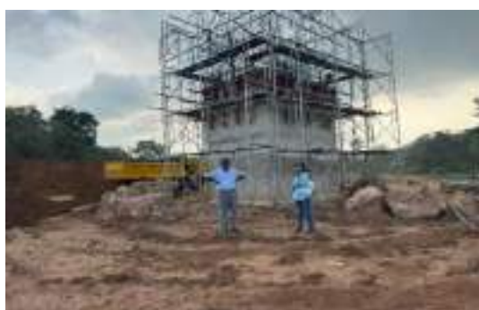
Figure 5-4: Construction of Sluice tower
