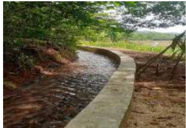
Figure 11-51: Rehabilitation of Karabalketiya Canal and Retaining wall (80m) at Wewathenna
