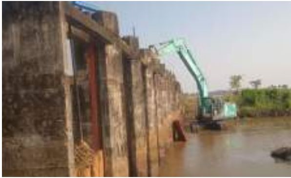
Figure 11-69: Supplying and installing steel gate with component to Vellaviralodai anicut in Rugam
