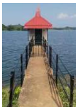
Figure 11-35: Improvements to RB and LB sluice houses in Dambarawa Scheme / Head Works
