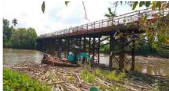
Figure 11-87: Clearing obstacles at Wakwella bridge
