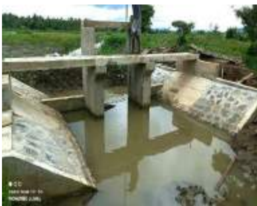
Figure 11-182: Providing 600mm Dia pipe inlet & outlet for Kankunwela pooling section & from the feeder canal bund from 2+500 to 2+950m in Wanela scheme
