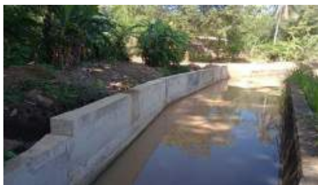
Figure 11-124: 2+250 Canal construction works
