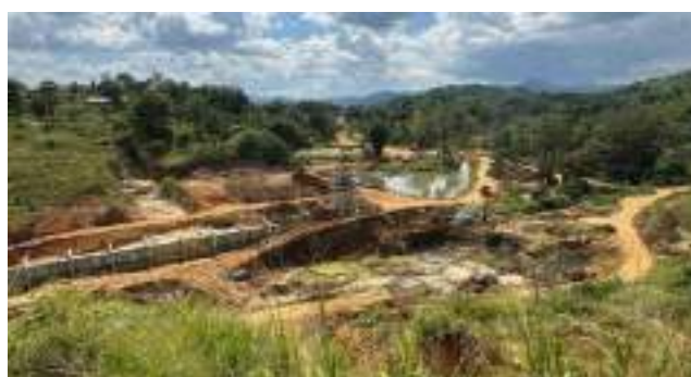
Figure 5-5: Sluice structure and Right Bank of Main Bund
