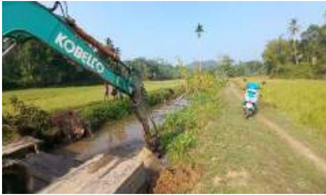
Figure 7-13: Clearing Nape main canal 3+270 to 4+210 & 6+310 to 8+750km at Kadduwa Scheme
