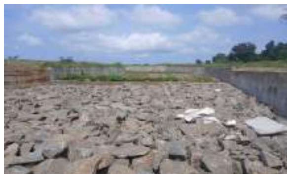
Figure 11-149: Improvements to Viyadikulam spill tail canal
