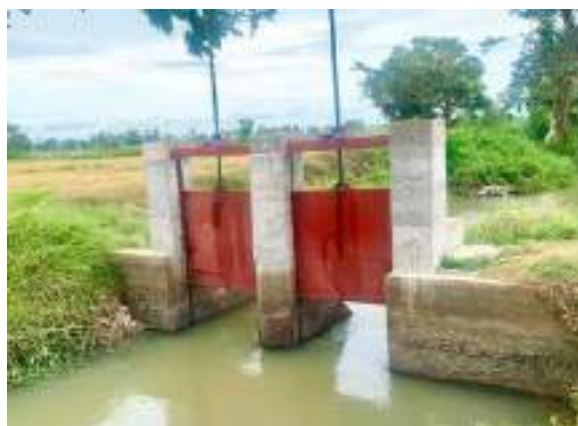
Figure 11-68: Providing gate arrangement to Mangalamadu offtake in Rugam scheme Division
