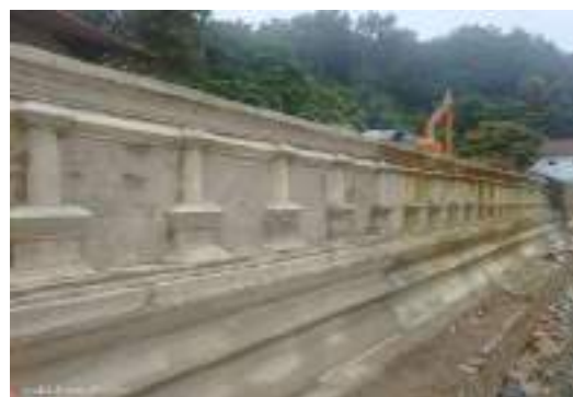
Figure 6-19: Construction of collapsed retaining Wall in front of Wishnu Dewalaya at Dalada Maligawa Premises in Kandy Region
