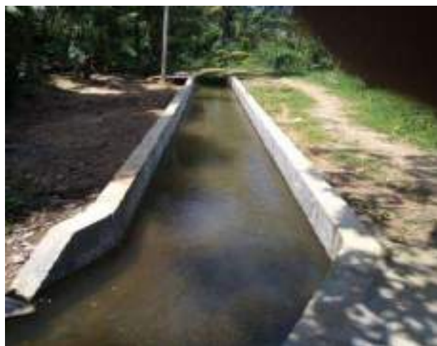
Figure 11-114: Construction of 15 m canal lining at 1+330 & 12m construction lining at 1+400 in main canal in Mulhal ela
