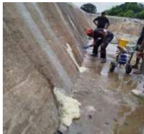
Figure 11-169: Improvements to Spill Structure 1 st Stage in Pahariya Scheme
