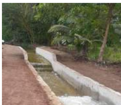
Figure 11-19: Con. of Drainage under crossing structure including drop Structure at CH 1+089 km at Solewewa Feeder canal LB tr.04
