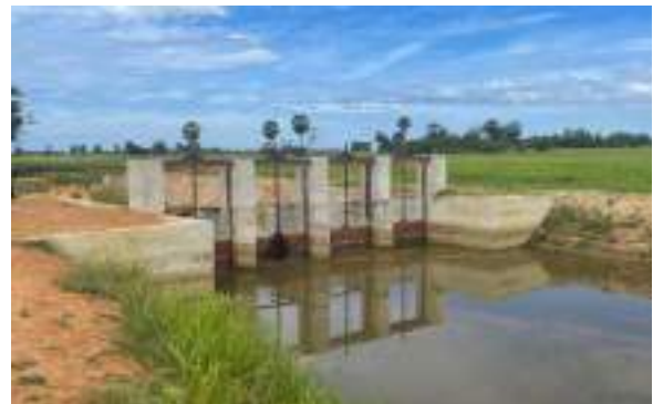
Figure 11-74: Re-construction of Vinayakar Anicut in Nawakiri Division
