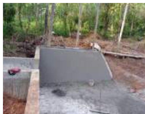
Figure 11-125: +100 Retaining wall construction
