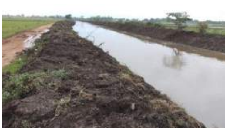
Figure 11-188: Desilting work in Helaba yaya to Egoda yaya drainage canal Stn 0+000 to Stn 2+200 in Janaranjana Scheme
