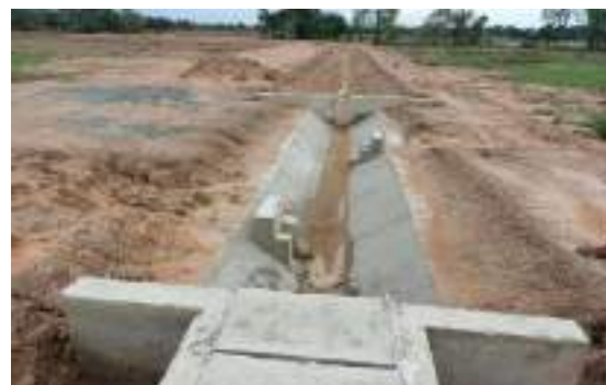
Figure 5-3: Issanwewa Irrigable Area development works
