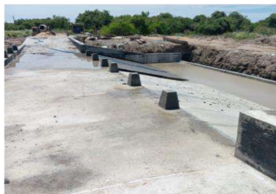
Figure 11-179: Construction of Spill - 03 Structure at 3+520 in Muthur Division, Trincomalee Region
