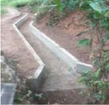
Figure 11-48: Concreting 6Km of Avukana canal in Uvathanna
