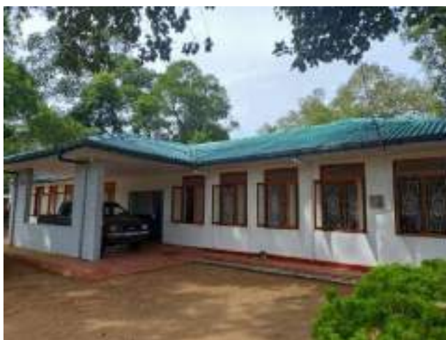
Figure 11-152: Improvements to DIE's office Building in Bibila Division
