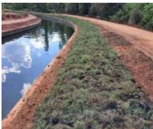
Figure 11-122: Construction of 150m long canal lining at 2+860
