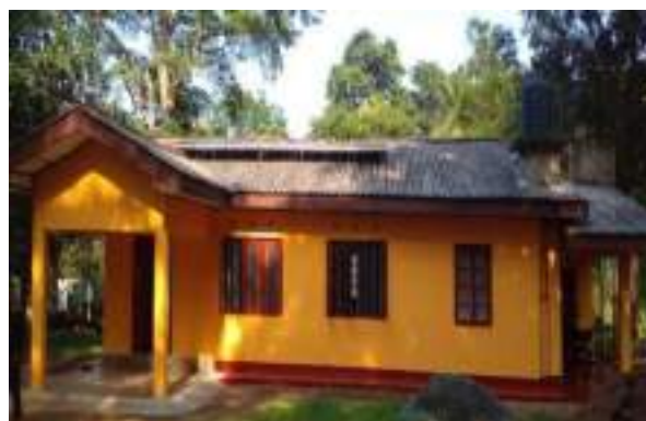
Figure 11-31: Rehabilitation of Sorabora unit office / Unit Office
