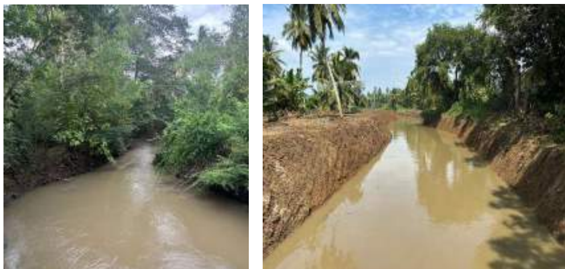
Figure 7-18: Canal widening, Desilting and clearing obstacles along Koggalu Ara in Hambantota division
