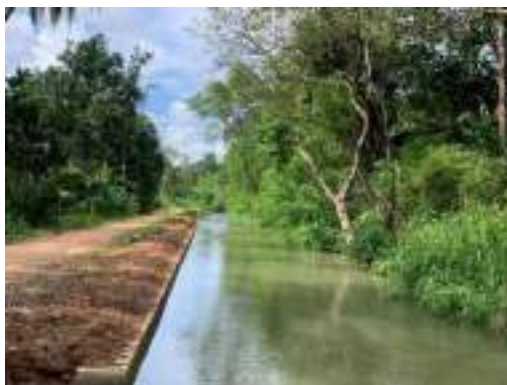
Figure 11-162: Construction of 14.7m retaining wall from 2+760 to 2+774, construction of 52.6m retaining wall from 2+776 to 2+828 in B 506/ B 507 in Elahara Division
