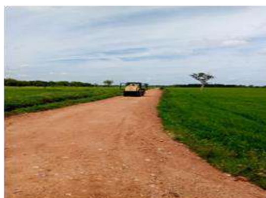
Figure 11-181: Improvements to Sakalasooriya Yaya Road from 0+000 to 0+925 in Janaranjana Scheme, Kantale Division
