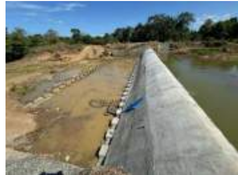
Figure 11-177: Raising of Savararu Anicut crest level in Morawewa Scheme
