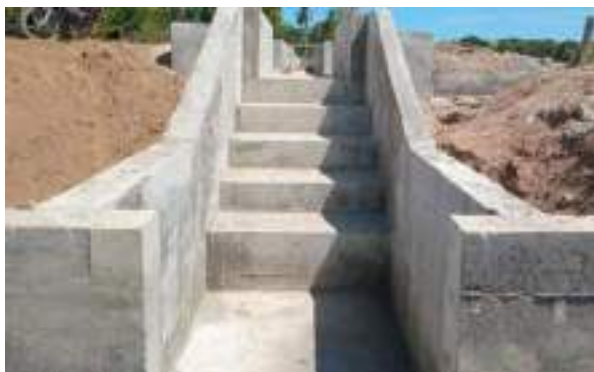
Figure 11-59: Improvement to LB -36-D channel from stn 0+350 to Stn 0+530 in Navakiri scheme
