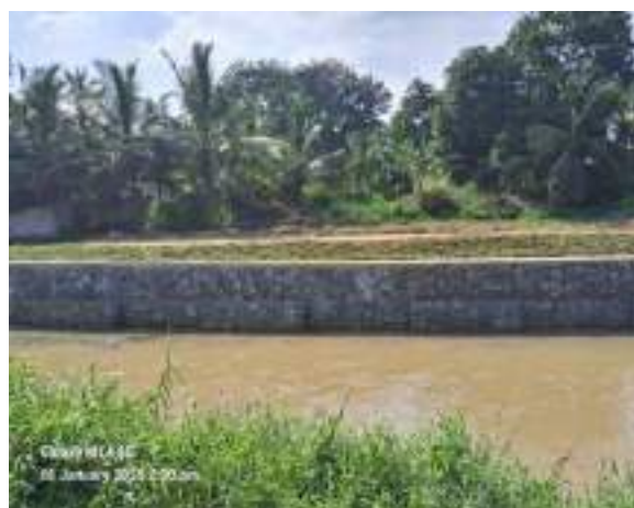
Figure 11-96: Construction of protection wall for Kirama oya RB side at downstream of Danketiya anicut in Kirama oya scheme
