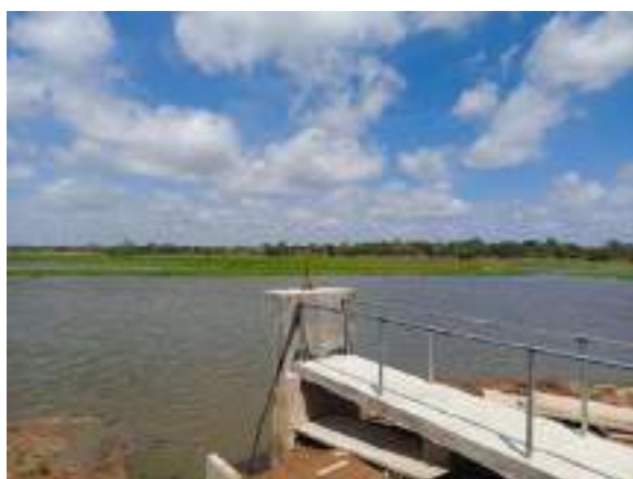
Figure 11-18: Repairs to Thirappankadawala LB sluice
