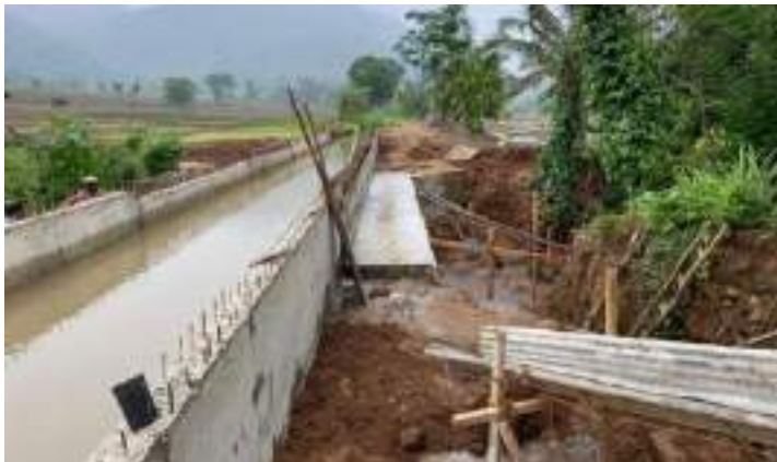
Figure 11-52: - Construction of Trough at 1+615 of Meda ela in Bathmedilla scheme
