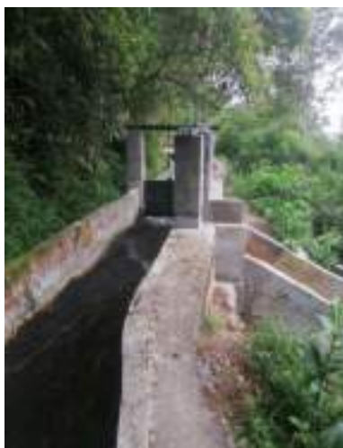
Figure 11-40: Construction of spill gate at 0+744Km in Kande ela Scheme / FDR
