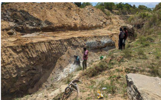
Figure 11-63: Improvements to Muruthanai offtake channel in Punanai scheme
