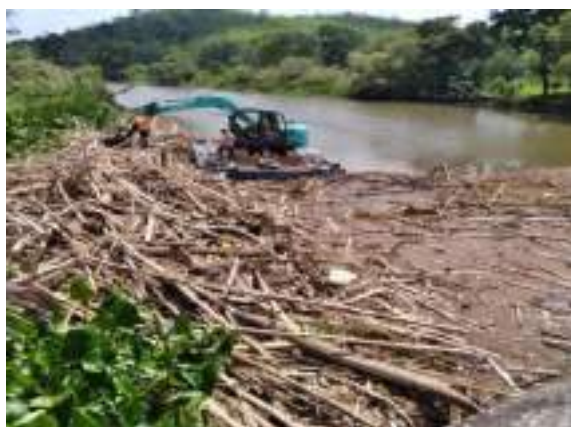
Figure 11-90: Clearing obstacles at Awitthawa bridge in Ambalangoda division
