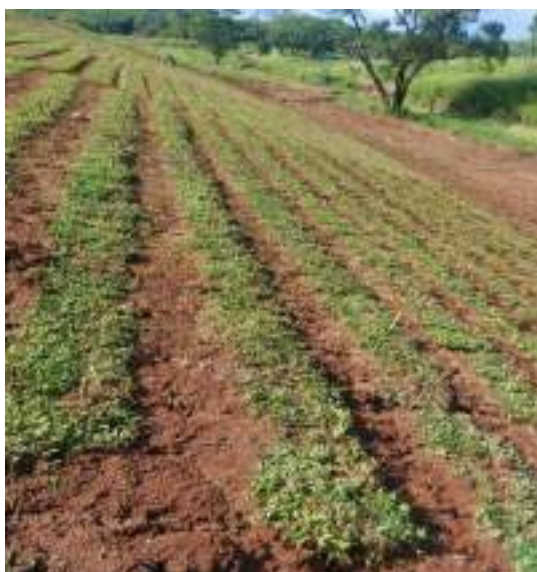
Figure 11-108: Improvement to D/S of tank bund and Turfing
