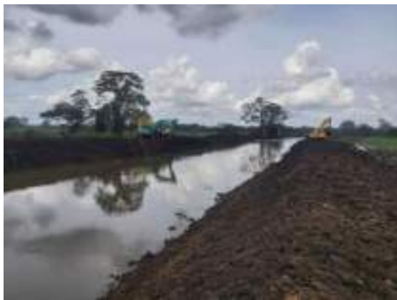
Figure 6-16: Kaudulla spill tail canal widening from 29+540 to 30+400
