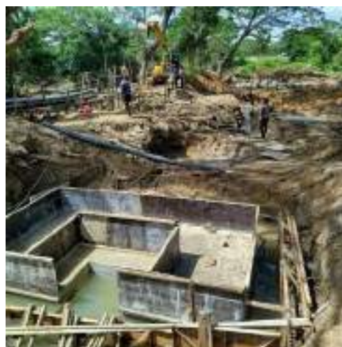
Figure 11-174: Removing of Damaged Trough Structure and Construction of New One at 1 st km in LBMC in Kottukachchiya Scheme
