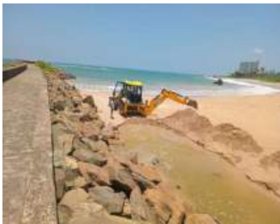
Figure 11-88: Widening of Kapu Ela sea outlet at Mahamodara
