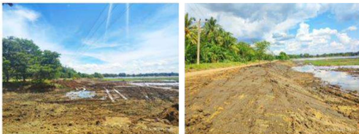
Figure 11-164: Removing sediment materials at Kadawalawawa tank LB entrance in Girithale scheme in Minneriya division
