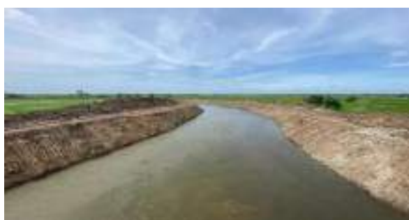
Figure 7-1: -Open the Kantale reservoir Spill tail canal bend section at 15+000 and strength the bund in Kantale Division in Trincomalee Region
