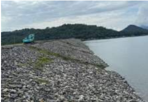
Figure 11-2: Providing of Rip-Rap Protection to Senanayaka Samudraya Bund and Improvements to Bund Road under IWWRMP
