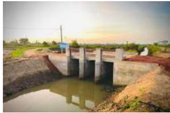
Figure 11-72: Improvements to Pandarakkadu bridge cum regulator in Rugam Scheme,
