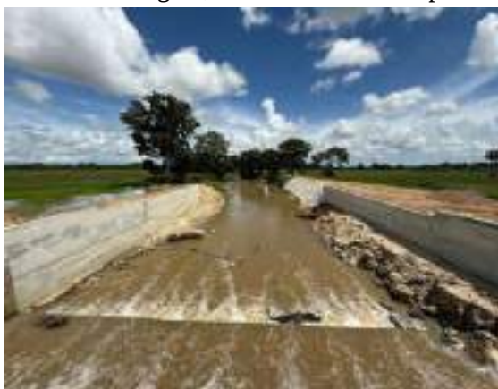
Figure 7-4: Improvements to RB downstream protection in Kalvaddai Anicut in Navakiri scheme in Navakiri Division in Batticaloa Region
