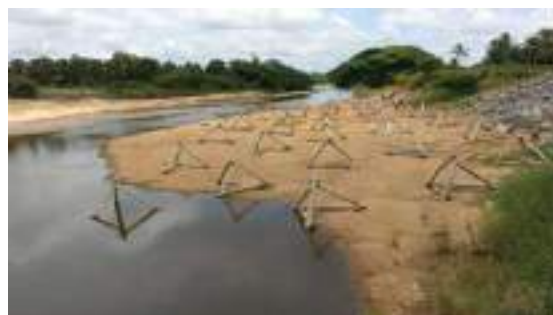
Figure 7-2: Protection of Sengaloya anicut RB side in using RCC procupine structures in Puttalam Region
