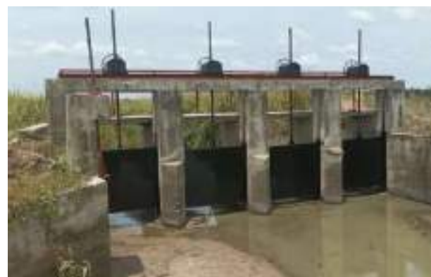
Figure 11-7: Improvements to Damanayaya Anicut in Lahugala scheme in Pottuvil Division
