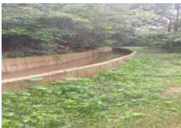
Figure 11-38: Construction of canal lining at 11+600 in main canal in Komarika ela scheme / ERMMS
