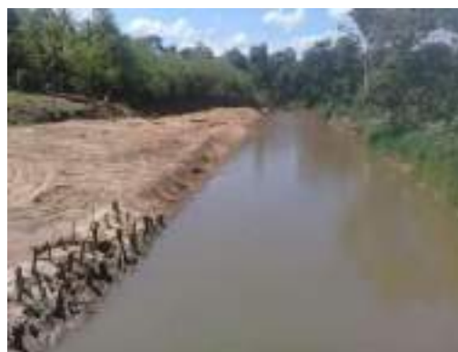
Figure 11-156: Embankment protection of river bank by providing timber piles in Galoya river in Bibila Division
