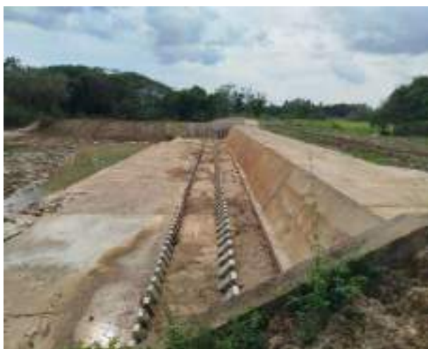
Figure 11-173: Improvements to Maiyawa Tank and 1 st Spill in Sengal Oya Scheme
