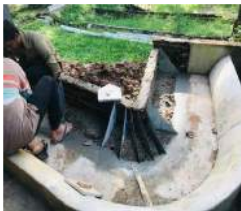
Figure 4-13: Modification works of Ellewewa uncontrolled chute spillway
