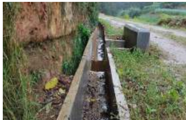
Figure 5-15: Construction drainage inlet
