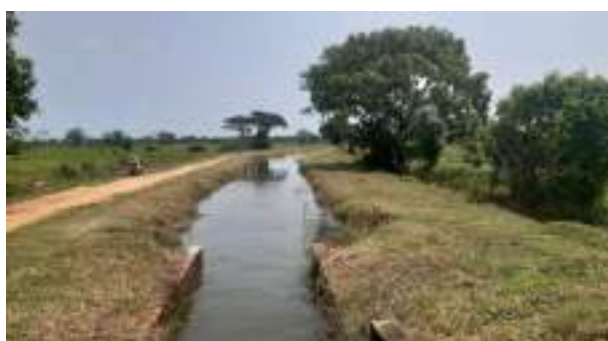
Figure 11-147: O &M works at Akathimurippu
