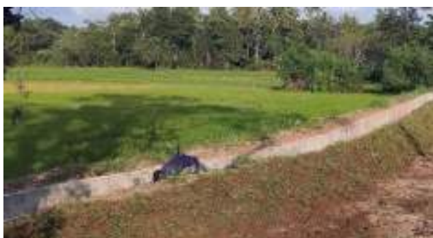
Figure 11-158: Construction of 90 m long rectangular canal lining from 0+475 to 0+565 in track 40 DFC canal in Ihakuluwewa FO area in Elahera division
