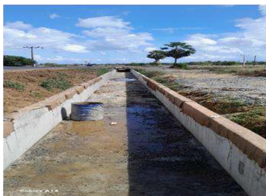
Figure 11-180: Construction of canal lining from 4+950 to 5+460 in Muthur Canal D06/LBMC in Muthur Division
