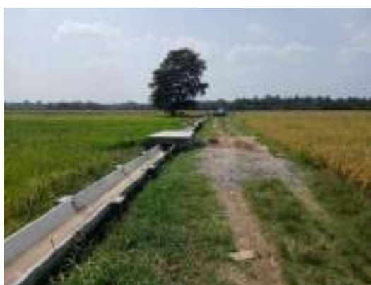
Figure 11-142: Half Round Canal System at Wellangiriya
