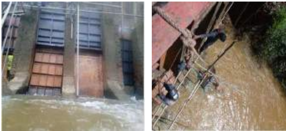
Figure 8-7: Hanpita Flood Gate repair by Central Workshop Rathmalana
