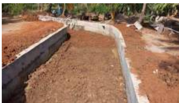
Figure 11-33: Construction of Retaining walls of 25m,21m and 20m long at 3+840 in RBMC in Mapakada Scheme / FDR
