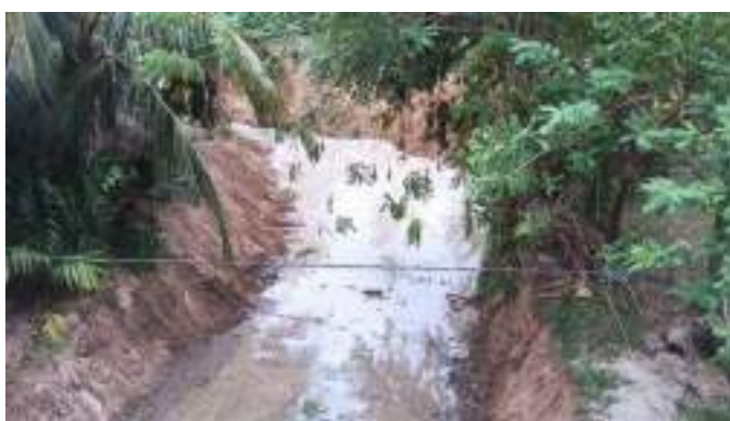
Figure 11-155: Clearing Kumbukkana oya river U/S & D/S anicuts & Makul Ara stream in Monaragala Division
