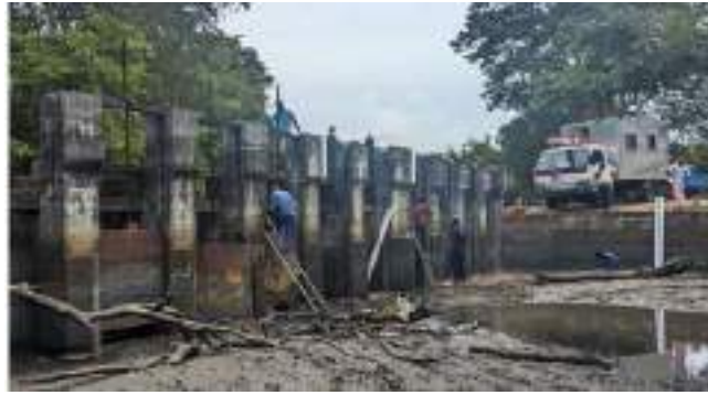
Figure 8-9: Mora Oya annicut gate Re Fabrication and Installation works by Regional Workshop Rambewa
