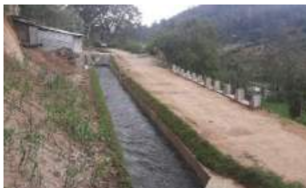
Figure 6-21: Construction of 72m long canal lining at 1+500 in Uma ela scheme in Mannar Region
