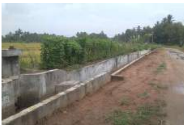
Figure 11-160: Re-construction of D37 canal lining from 6+255 to 6+317 under PIDP in Minneriya division
