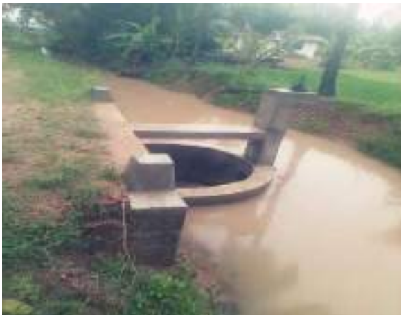
Figure 11-4: Improvements of structures in G 07 canal at Gonagolla Unit Ampara division
