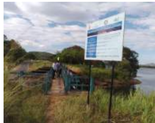
Figure 6-23: Nagadeepa Tank bund, spill way and improvement progress of the bund in Mapakada Division – Badulla Region
