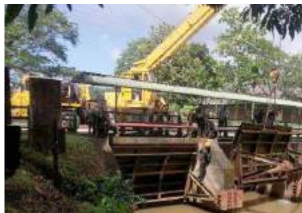
Figure 11-91: Repair works of Magallagoda gravity radial gates.
