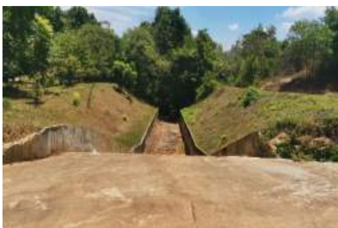
Figure 11-34: Improvements to spill in Dambarawa Scheme / Head Works
