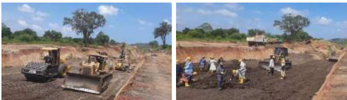
Figure 5-8: Construction works of Lower Malwathu oya Project
