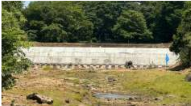
Figure 11-177: Raising of Savararu Anicut crest level in Morawewa Scheme
