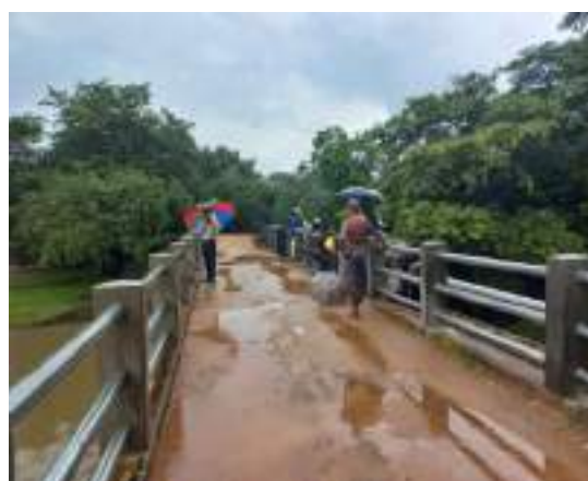
Figure 11-22: Improvements to handrail in Illukwewa Anicut to increase safety, Huruluwewa Division
