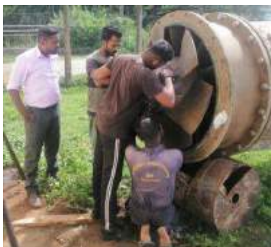
Figure 11-92: Repair works of axial flow pumps of Nilwala pump houses
