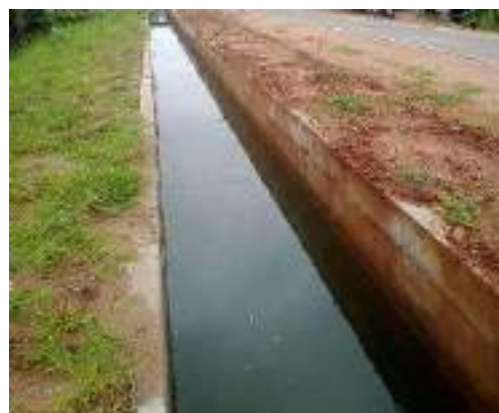
Figure 11-161: Construction of rectangular canal lining from 2+525 to 2+710 in LBMC in Ambagaswewa tank in Kaudulla Division
