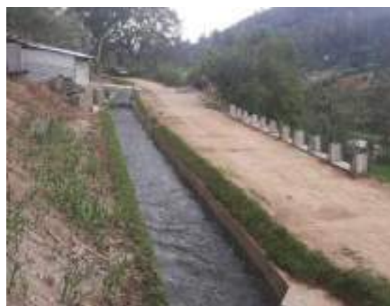
Figure 11-42: Construction of 72m long canal lining with construction of 15m long gabion toe wall at 1+500 Uma ela Scheme / ERMMS
