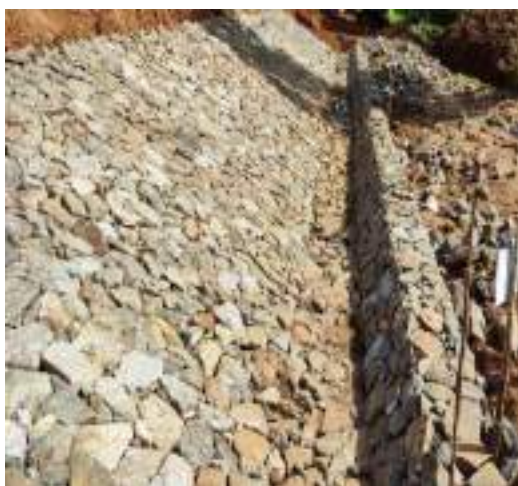
Figure 5-12: Construction of toe filter
