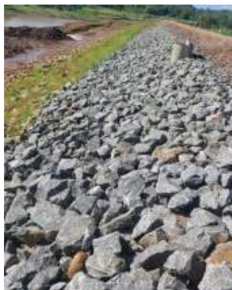
Figure 11-109: Replacing Rip-rap
