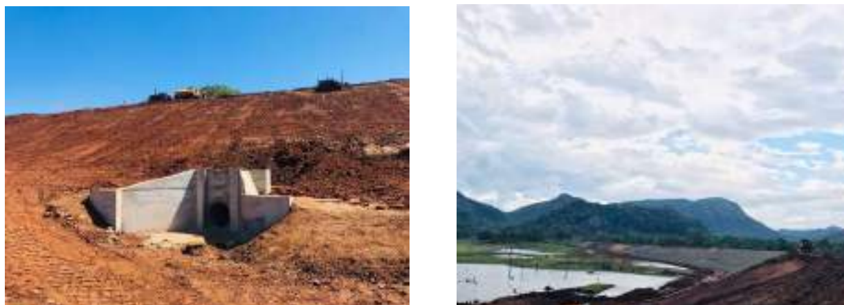
Figure 5-6: Upstream of Himbilyakada tank bund
