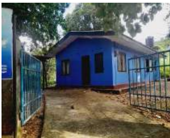
Figure 6-10: Improvements to Komarika Ela Unit Office in Kandekatiya
