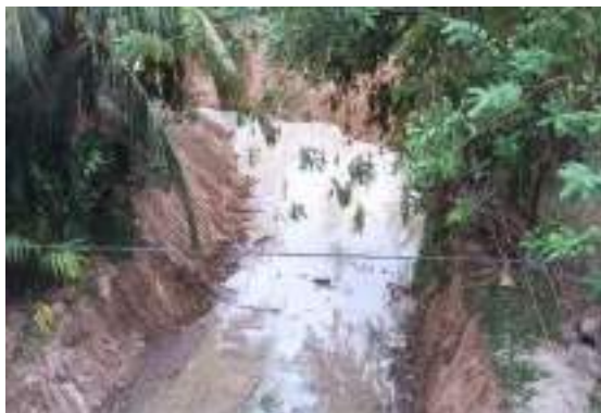
Figure 7-8: Clearing along Makulara Stream in Kumbukkana Scheme in Monaragala Region
