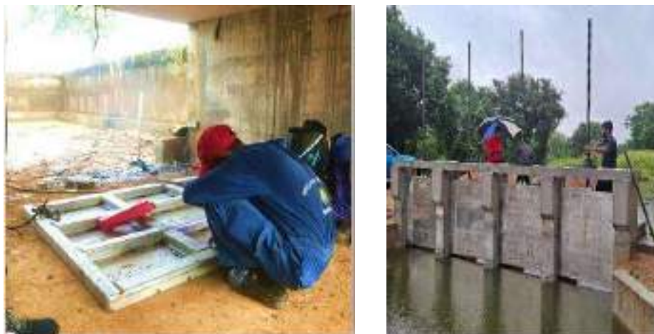
Figure 8-8: Eruwewa-Mahakanadarawa Feeder Canal Gate repair by Regional Mechanical Workshop Rambewa
