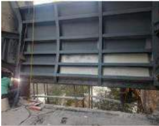
Figure 8-10: Mathalawewa Rotawewa Radial Gate Refabricates works by Regional workshop Minneriya
