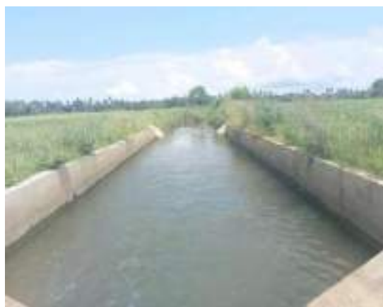
Figure 11-100: Improvements to Regulator at 2+186 in Kinchigune Main canal, Uruboku oya Scheme
