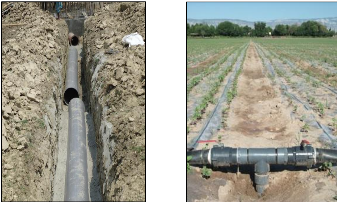
Figure 10: Sample images of the pipe alignment in the field.
